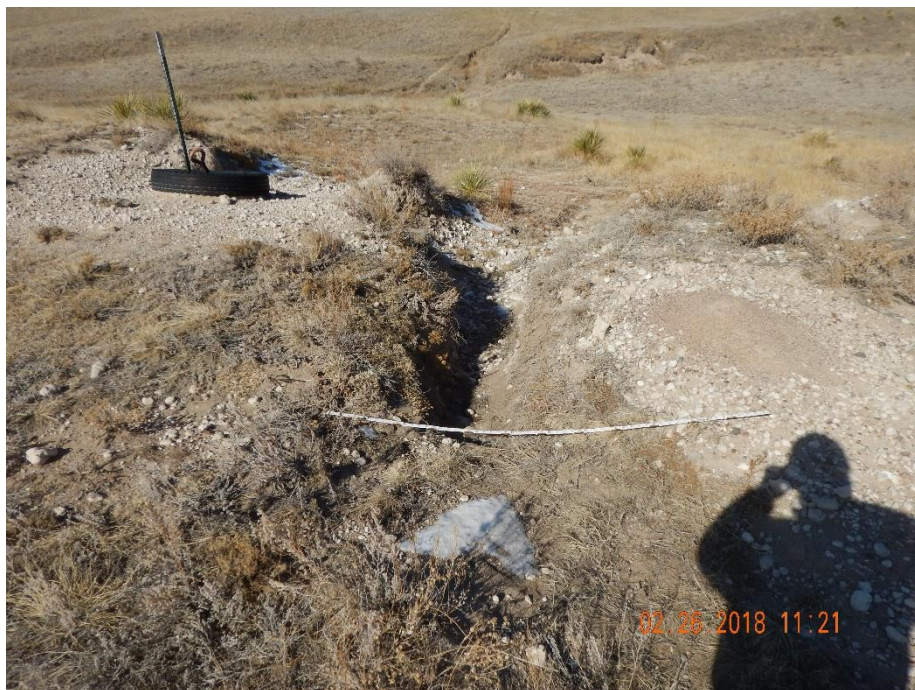
Photo 19: Photo taken from the west end of the location, facing west. Photo shows gully erosion due to stormwater erosion from the location has not been repaired, stabilized or reclaimed. No stabilization and stormwater BMPs have been installed or maintained. 6 foot measuring stick for reference.
