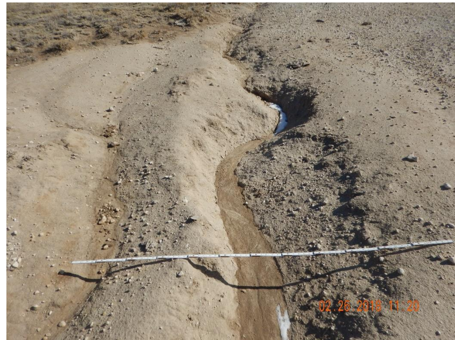
Photo 16: Photo taken from the southwest end of the location. Photo shows stormwater erosion degradation on the adjacent areas due to stormwater runoff from the location. See comments under photo 1.
