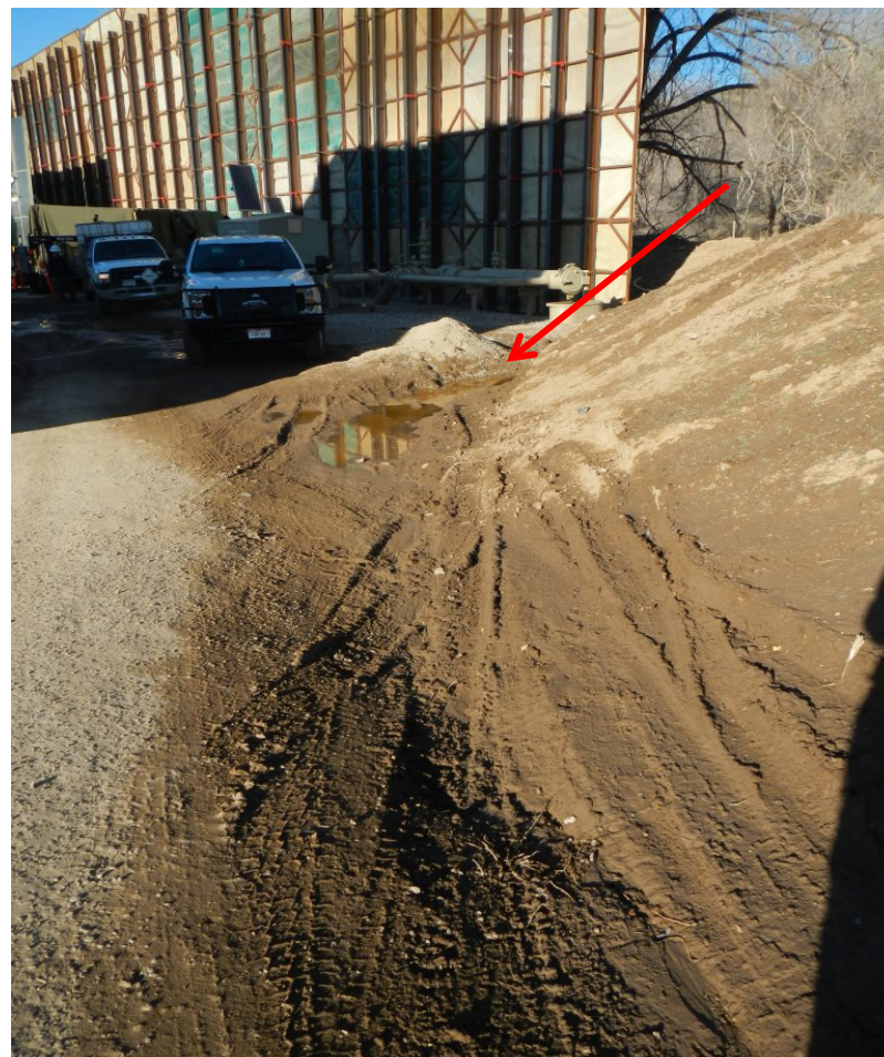
Photo#4: View South of Ditch on East side of Access Rd; arrow indicates spot where Material pile is blocking SW flow and Drain.
