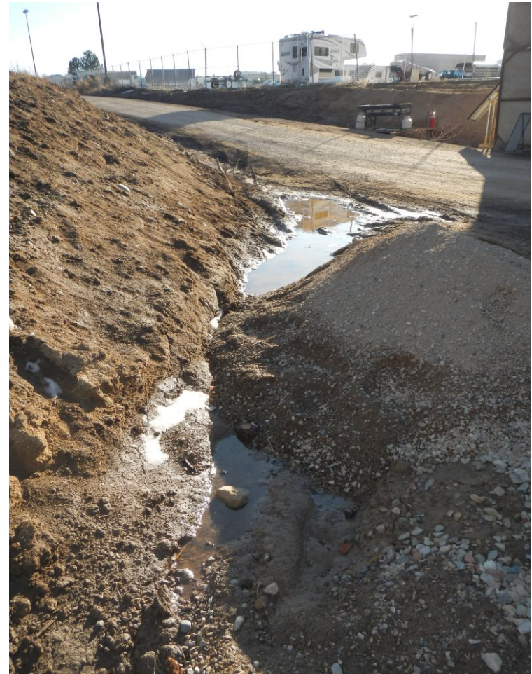
Photo#6: Looking back (Southwest) at blocked BMP
