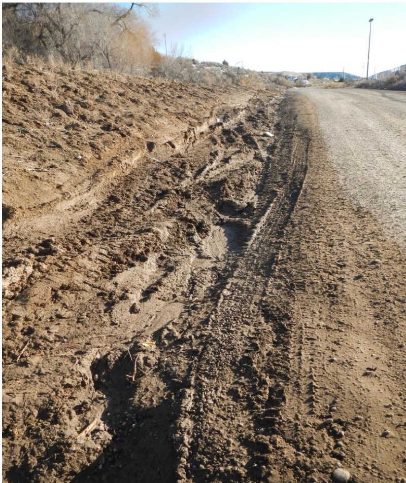
Photo#3: View South along ditch on East side of Access Rd; BMPs have been Compromised.
