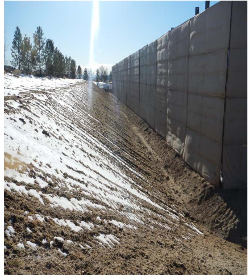
Photo#4: View along South Pad Perimeter & Sound Wall
