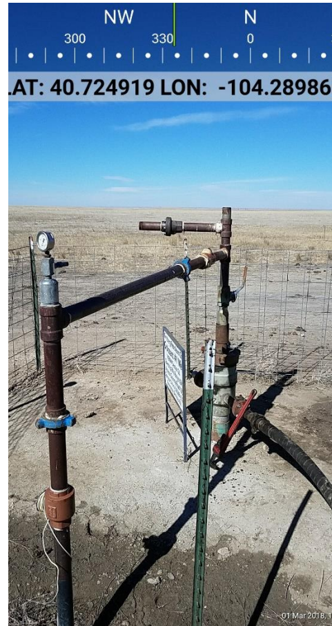
Photo 2 Current inspection photo, bradenhead not exposed at surface.
