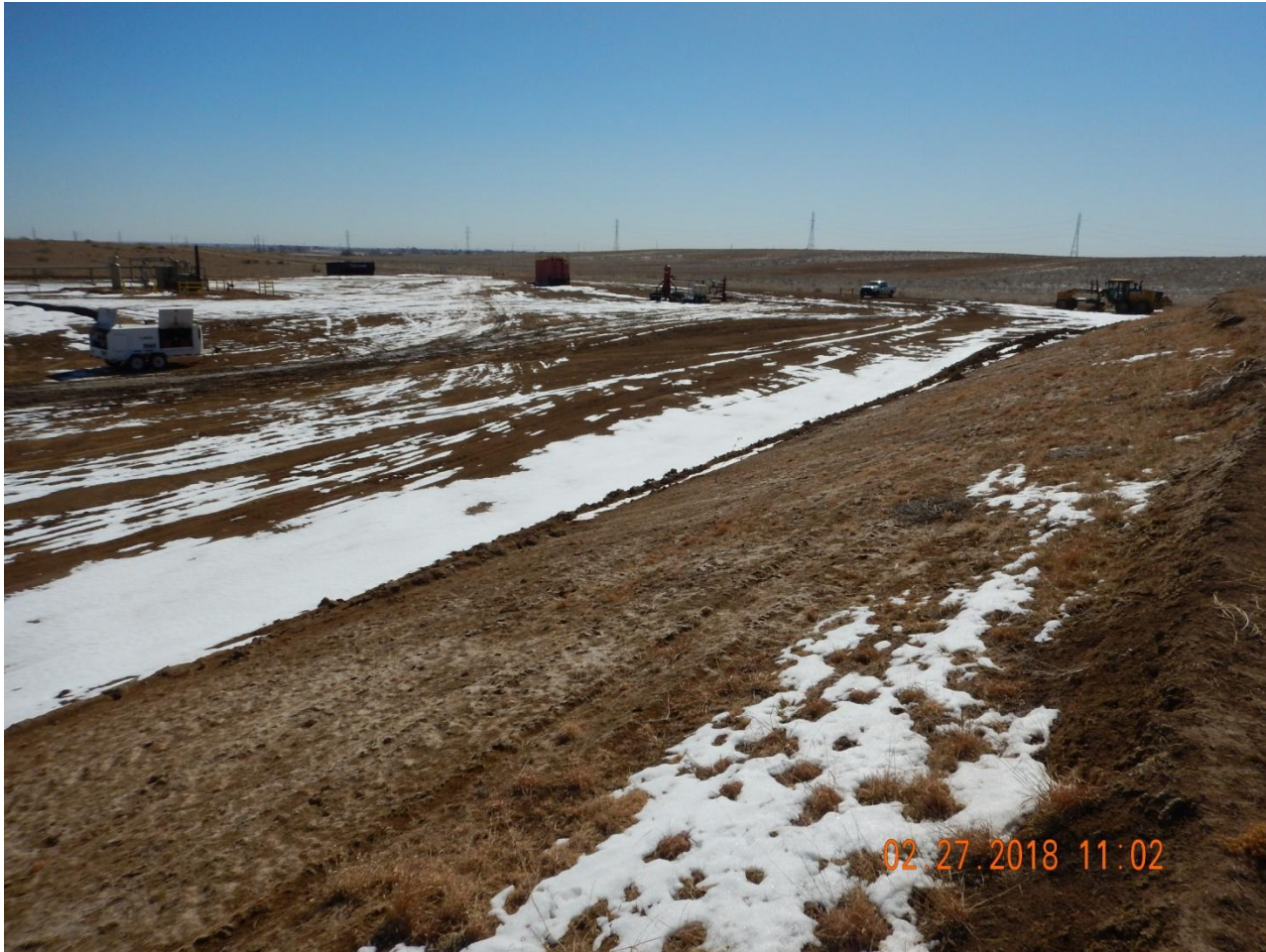
Photo 7. Photo taken from the western perimeter of the location, facing South. Operator has failed to perform interim reclamation to reduce areas not needed for production operations per Rule 1003.
