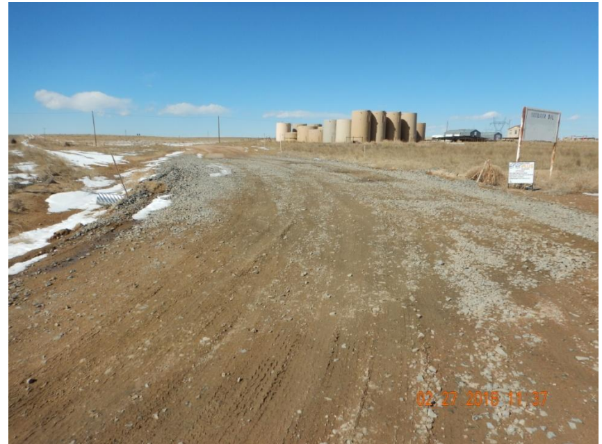
Photo 2. Photo taken from the entrance of the location off the intersection of CR 25 & CR 86, facing West. Operator has installed a tracking pad device. Appears maintenance may be needed for the tracking pad.
