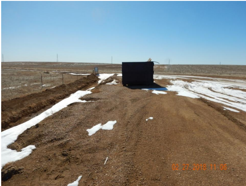
Photo 5. Photo taken near the entrance of the well pad location, facing South. Operator has a trash bin at location which is not covered- see Photo 6.
