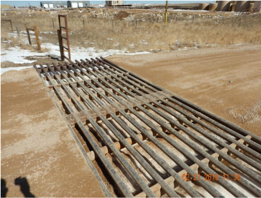
Photo 3. Photo taken of another tracking pad device along the eastern main access road, facing North. Tracking pad device appears to be proper functioning condition.
