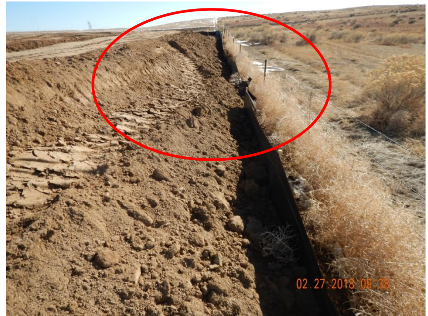
Photo 6. Photo taken from the southern perimeter of the location, facing East. Silt fence BMP has been damaged from topsoil storage operations. Operator representative at location indicated the BMP was scheduled to be fixed sometime on February 27, 2018.
