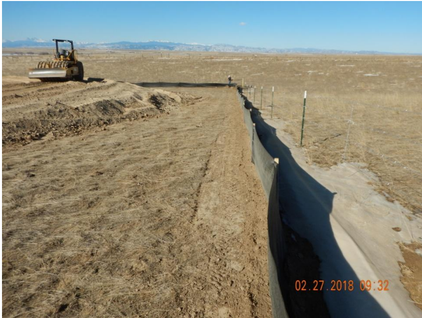
Photo 3. Photo taken from the northwest perimeter of the location, facing West. Silt fence BMP has been installed around portions of the northern and eastern location, and the entire southern and western perimeter of the location.
