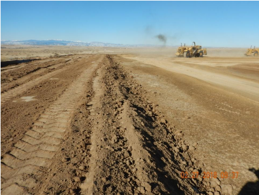
Photo 7. Photo taken from the southern location on the topsoil stockpile, facing West. Appears the Operator is still in-process of salvaging topsoil. Topsoil is being stored along the eastern and southern perimeter of the location.
