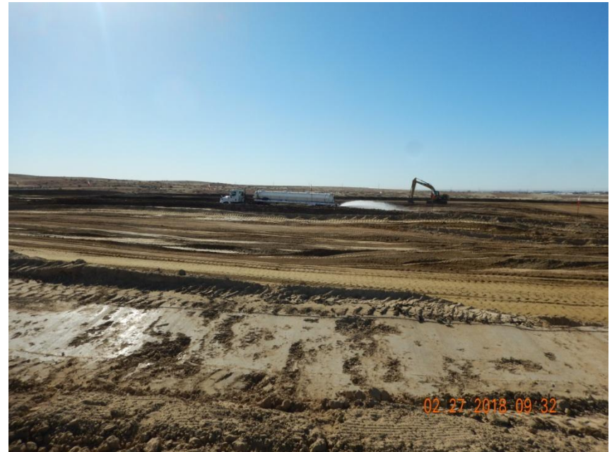
Photo 2. Photo taken from the northern perimeter of the location, facing South. Water truck at location to aid in construction operations and controlled fugitive dust.
