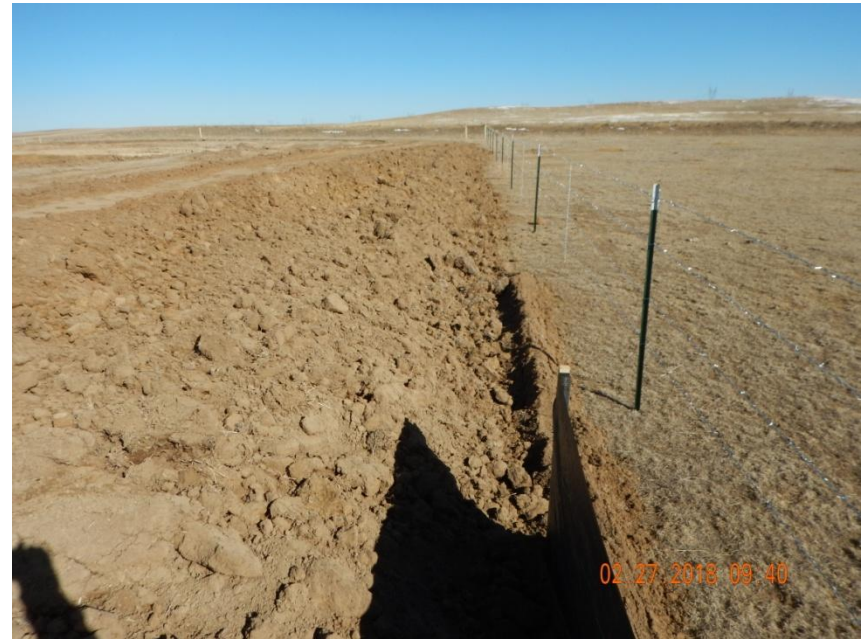
Photo 10. Photo taken from the eastern perimeter of the location, facing North. Silt fence BMP stops before the end of the topsoil stockpile. Operator shall install BMPs around all topsoil stockpiles. Operator representative at location indicated a BMP would be installed around the topsoil stockpile but did not provide a date.
