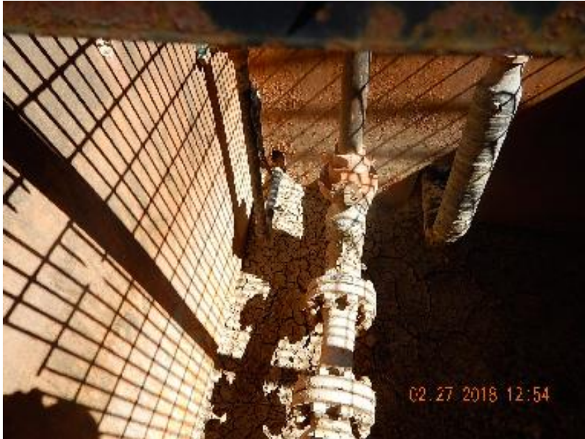
Photo 3: Unused 1" and 3" risers in #2 cellar.
