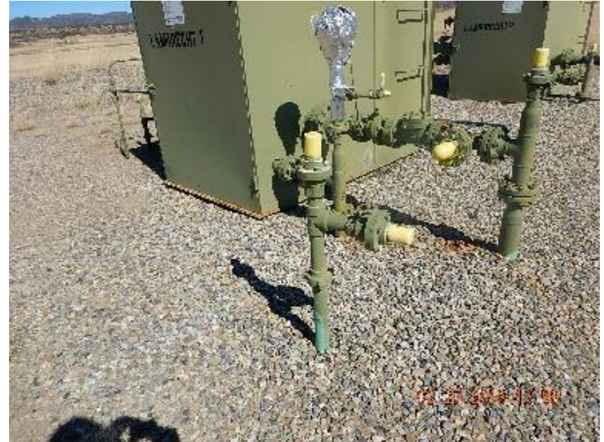
Photo 6: Unused 3" steel riser at separator.
