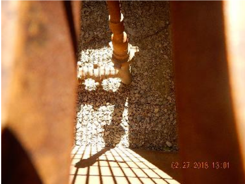
Photo 5: Unused 3" steel riser in #1 cellar.
