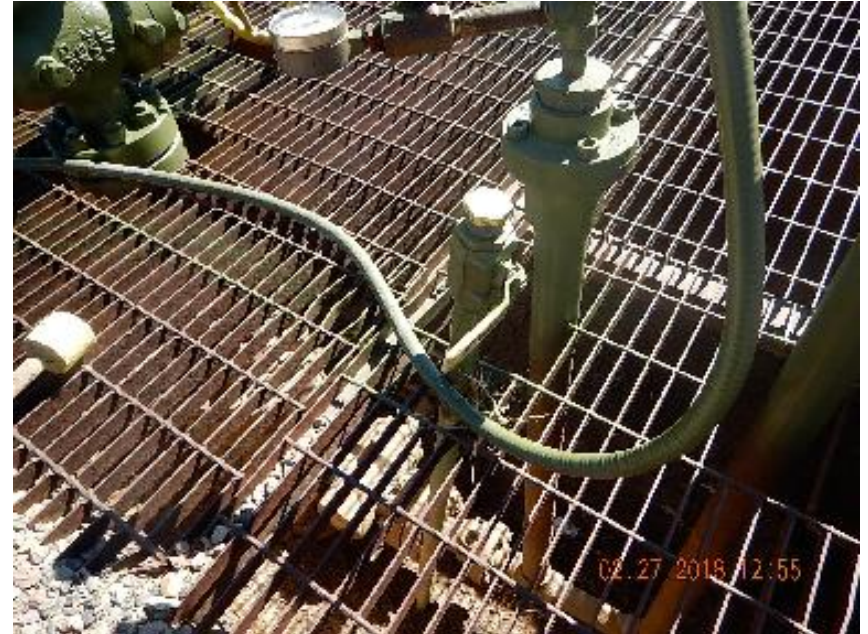
Photo 4: Unused 1" steel riser.
