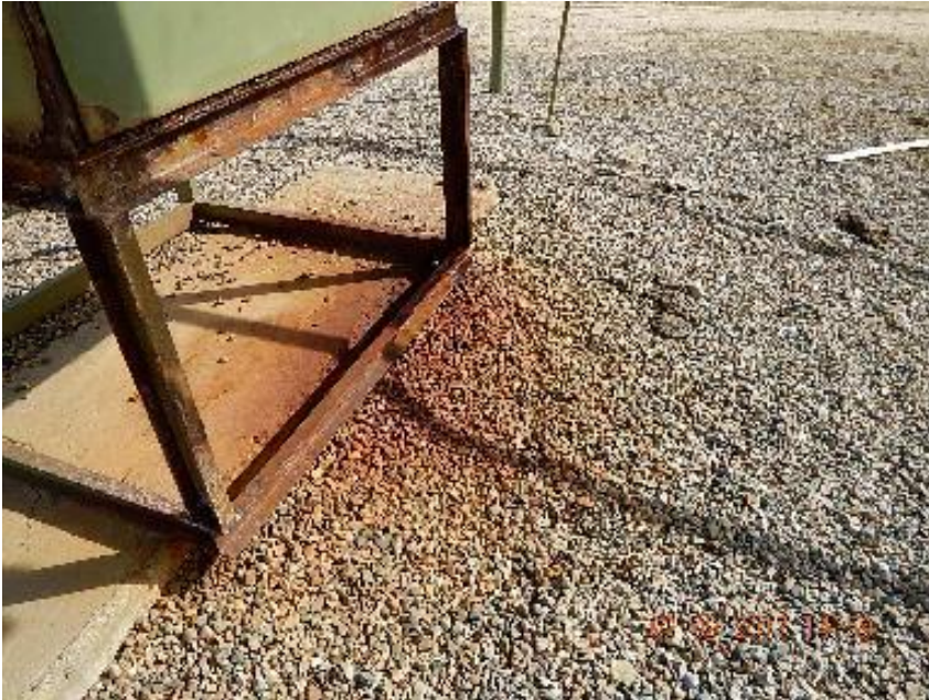
Photo 5: Stained soil and gravel under separator for Allison Unit Com #63 previous inspection.
