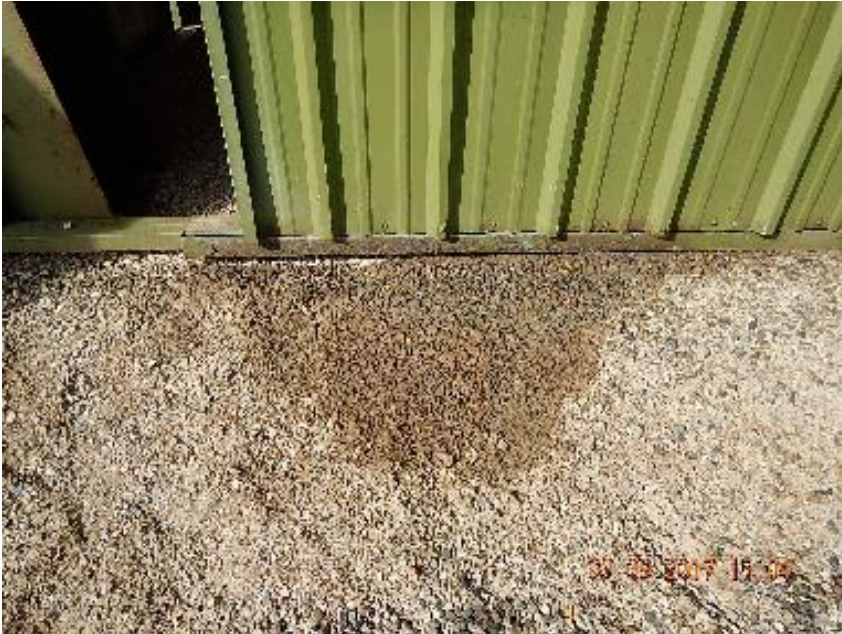
Photo 11: Impacted soil and gravel outside compressor entry noted in previous inspection.
