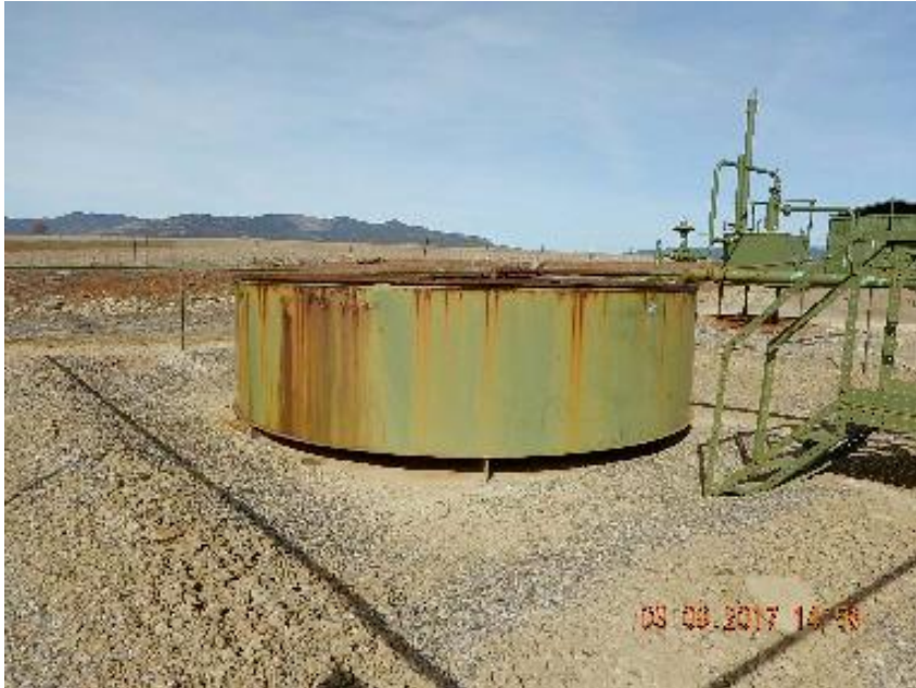
Photo 13: Rust streaked open top tank previous inspection.
