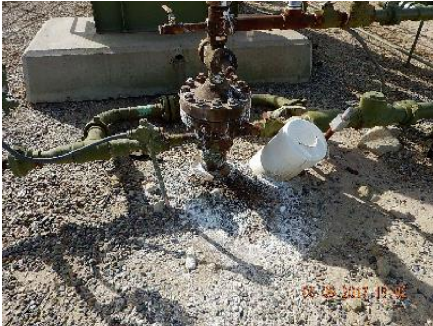
Photo 9: Impacted soil at wellhead previous inspection.
