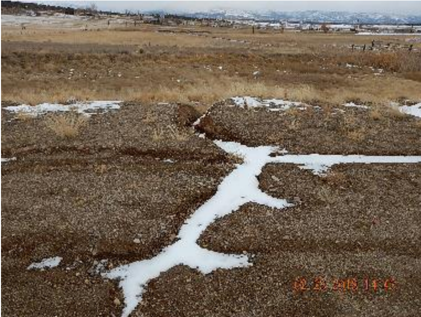
Photo 3: Erosion channel on E fill slope.
