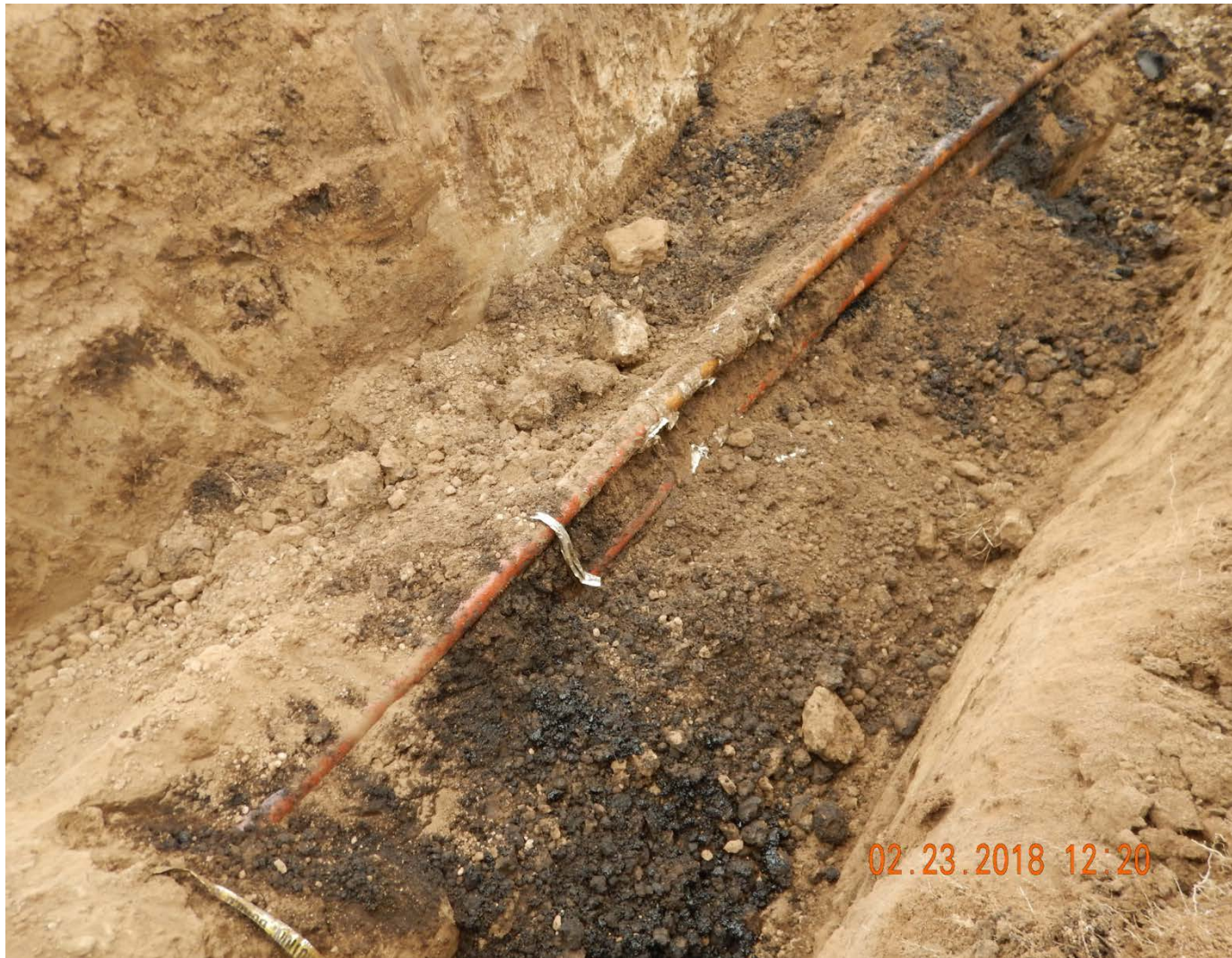
Pipeline excavation. Pipeline on top is source of leak.
