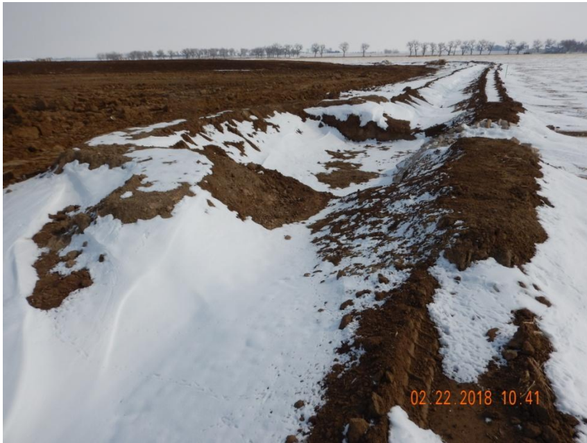
Photo 6. Photo taken from the southern location, facing East. Operator has installed a sediment trap in conjunction with the ditch and berm BMP.
