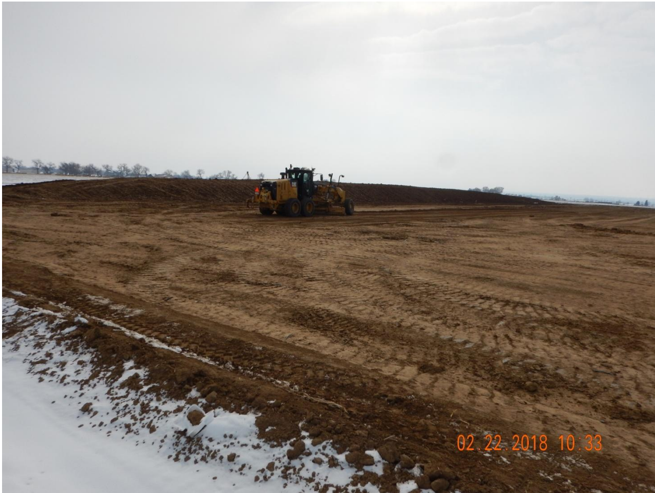
Photo 3. Photo taken from the northern location, facing Southeast. Appears topsoil has been salvaged and stored along the eastern perimeter of the location.
