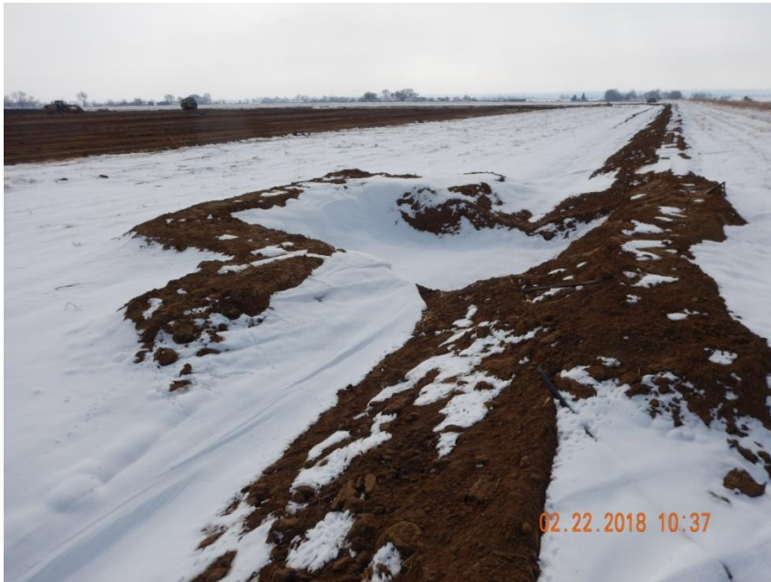
Photo 4. Photo taken from the western location, facing South. Operator has installed a retention area in conjunction with the ditch and berm BMP.
