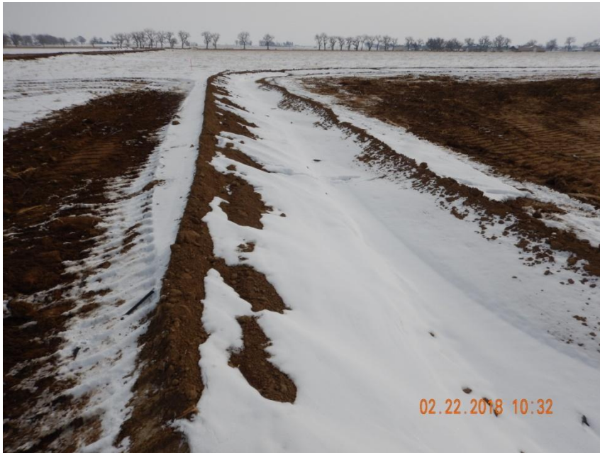
Photo 1. Photo taken from the northern location, facing East. Operator has installed a ditch and berm BMP around the perimeter of the location, in addition to retention areas and sediment traps.
