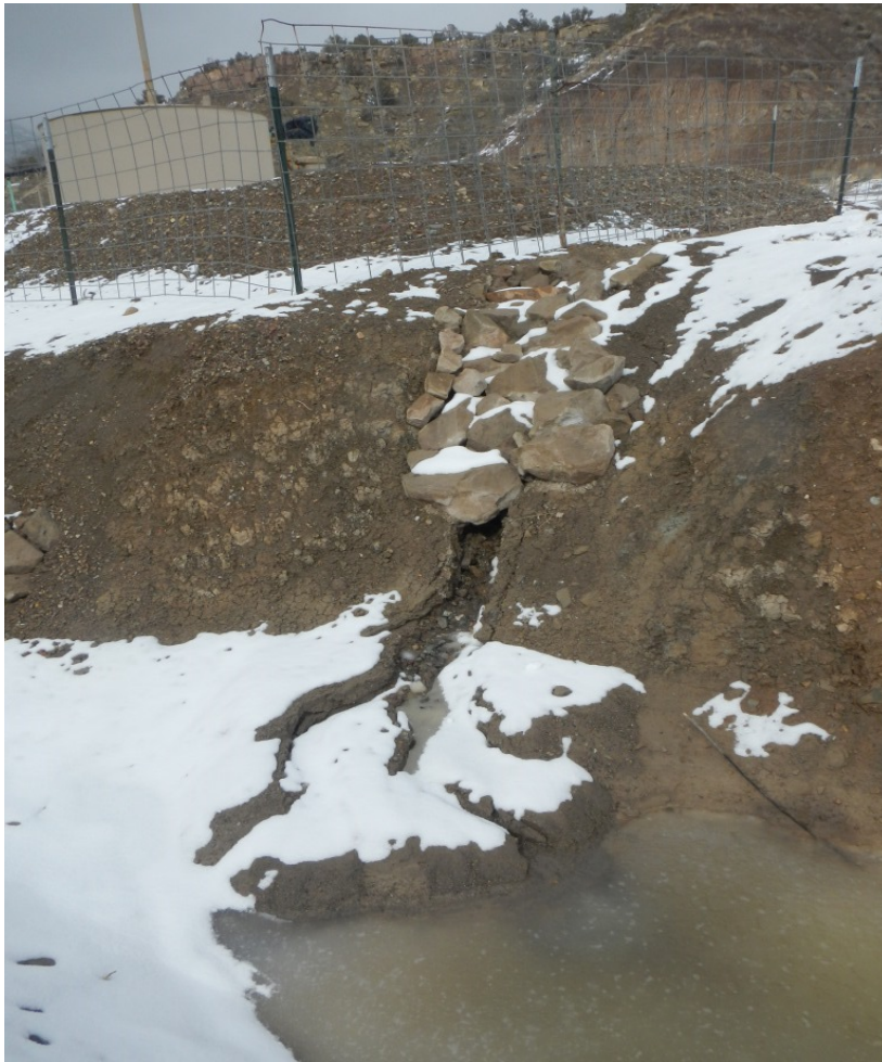
Photo#2: Storm water is Under cutting armoring/rip rap of drains into & out of Sediment traps.
