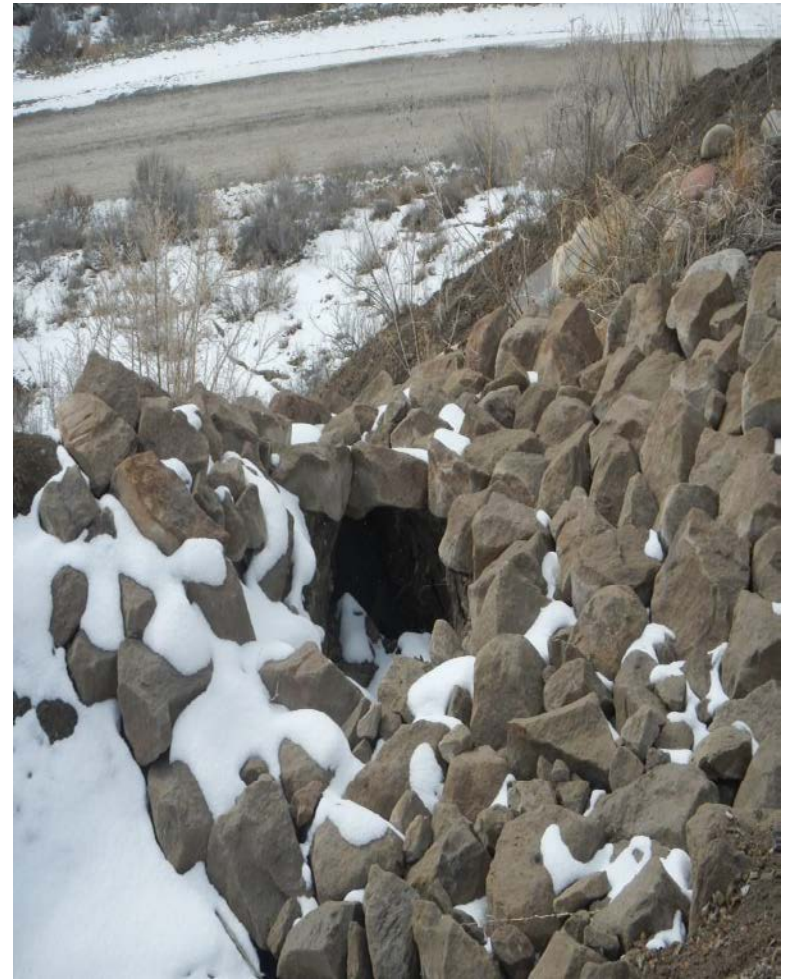
Photo#2: Storm water is Under cutting armoring/rip rap of drains into & out of Sediment traps.
