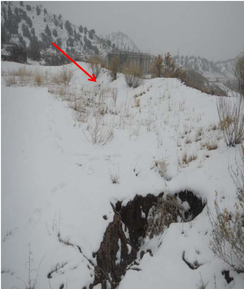
Photo#4: Subsidence in Ditch leading to Sediment Trap. Arrow indicates Sediment Trap.
