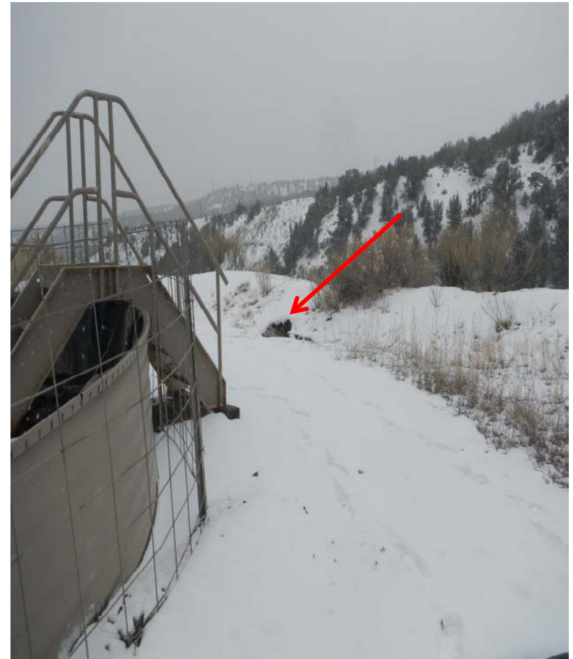
Photo#5: Position of Subsidence in relation to Tank Facility
