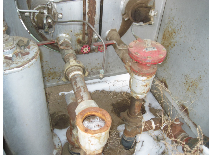
SOILED DIRT INSIDE SEPERATOR
