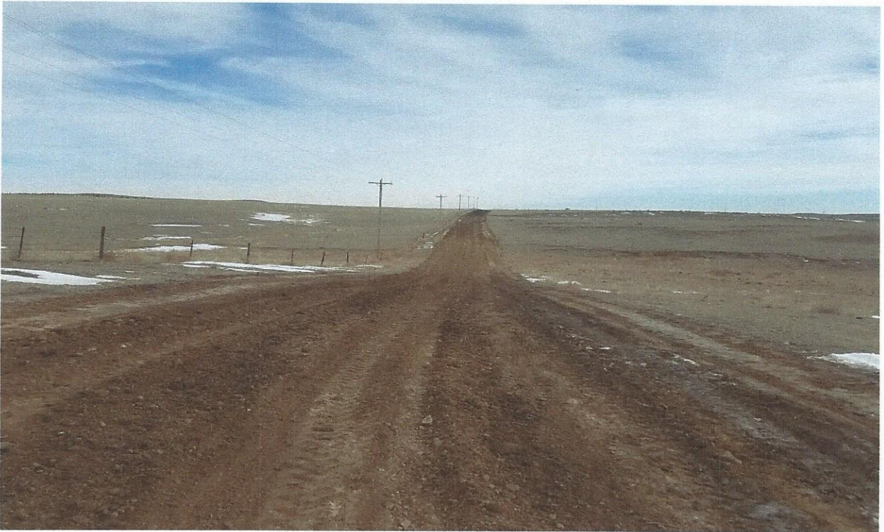
Main Access Road Ripped and Final Graded
