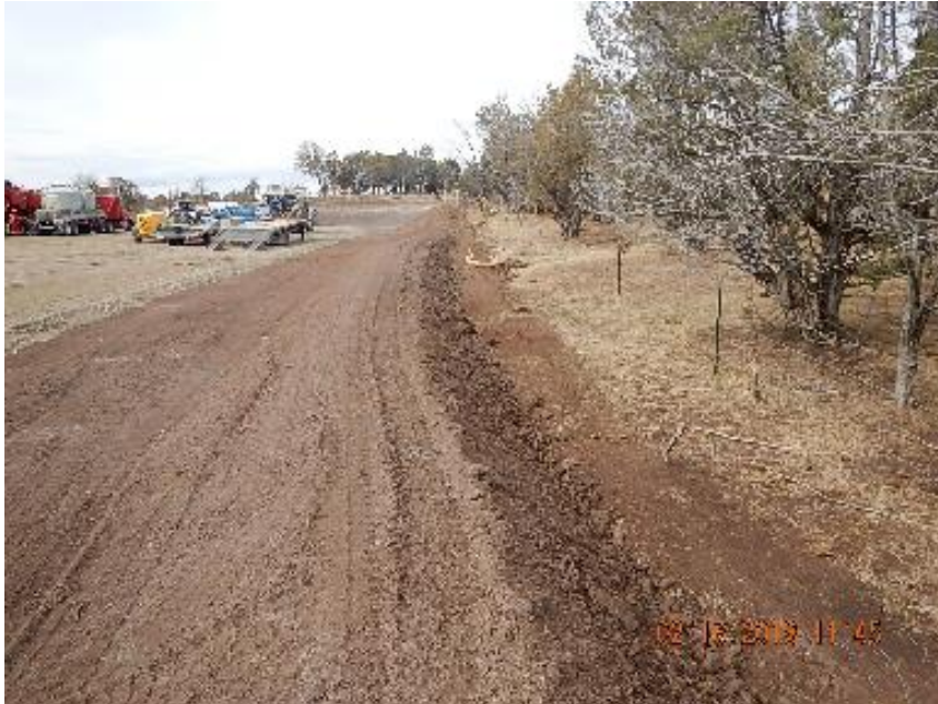
Photo 9: N perimeter looking NW. Berm and no erosion control waddle line. Single erosion control waddle check dam.
