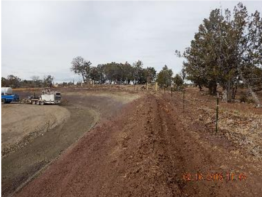
Photo 11: N perimeter approaching top of cut slope. Ditch and berm. No velocity control BMPs installed in ditch.
