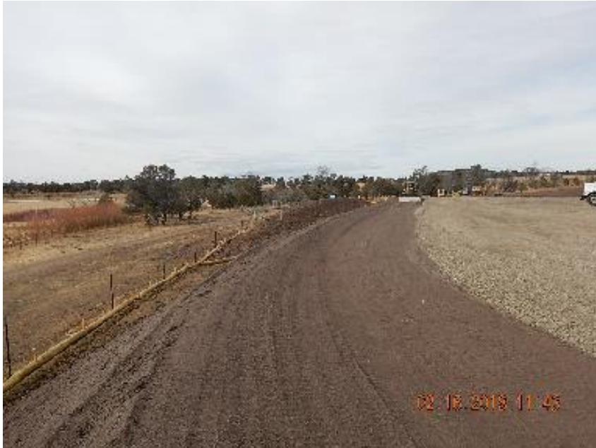
Photo 5: S perimeter looking NW. Waddles, berm, and edge of gravel not yet to base of berm.
