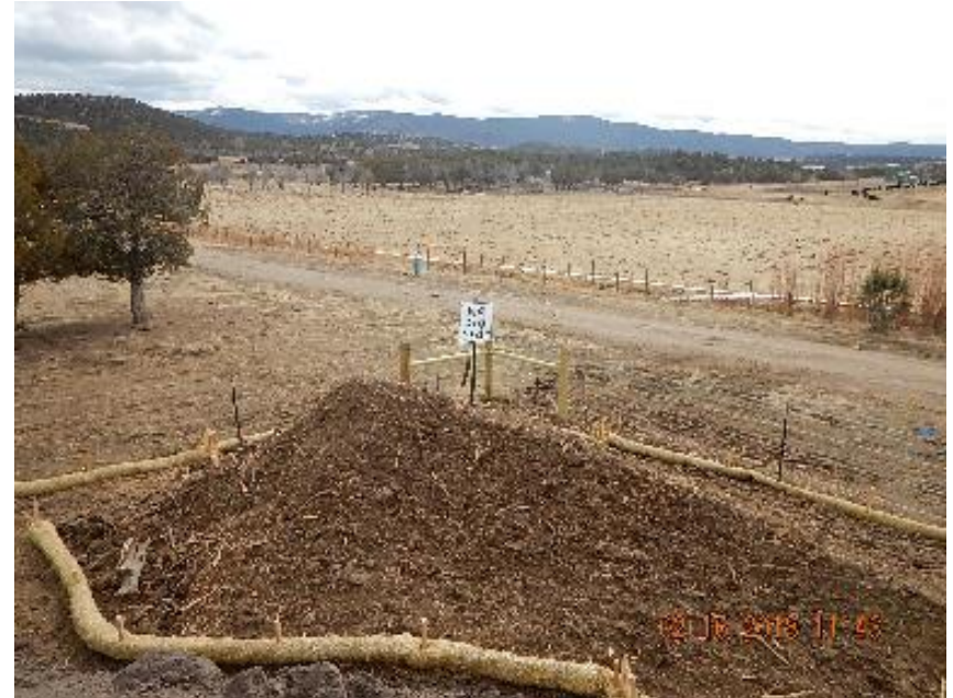
Photo 6: Additional top soil pile in SE corner with waddles and sign. Waddles improperly installed.
