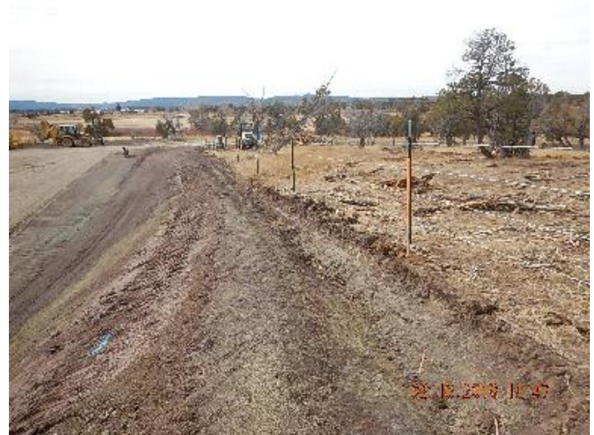
Photo 12: Top of cut slope looking S. Ditch and berm. No erosion control waddle line and no velocity control BMPs installed in ditch.
