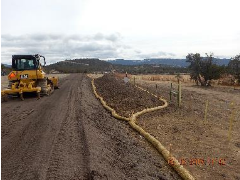
Photo 3: S perimeter looking E. Erosion control waddle and top soil pile along S perimeter. Waddle improperly installed.
