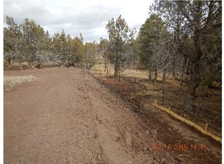
Photo 8: E perimeter with erosion control waddle line ending short of NE corner.
