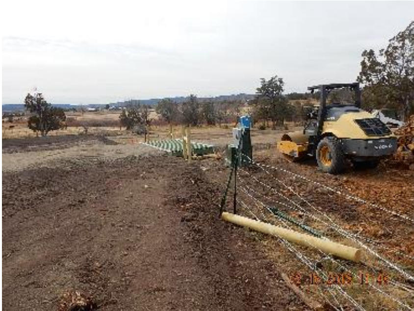
Photo 13: Cattle guard installed at entrance.
