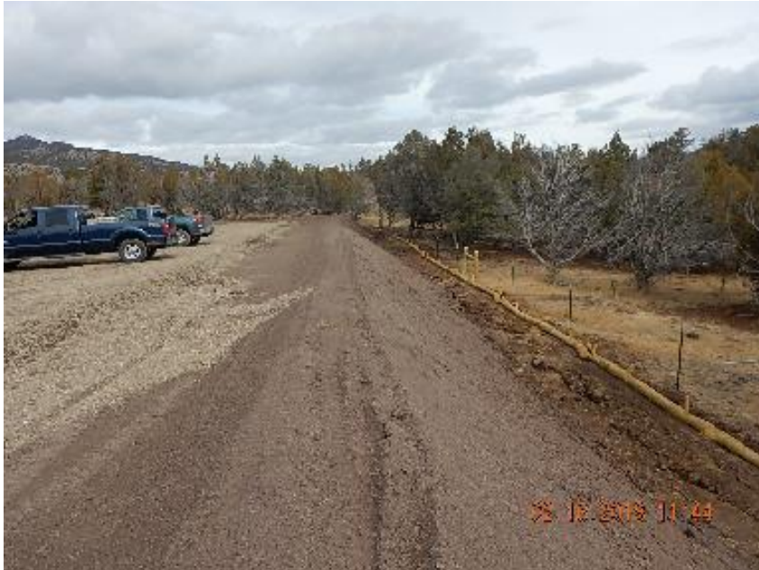
Photo 7: E perimeter looking N. Berm and erosion control waddles. Waddles improperly installed.
