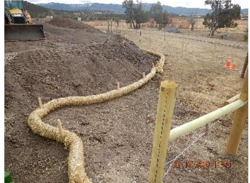
Photo 2: Erosion control waddle in SW corner not trenched in, not back filled, and improperly staked.
