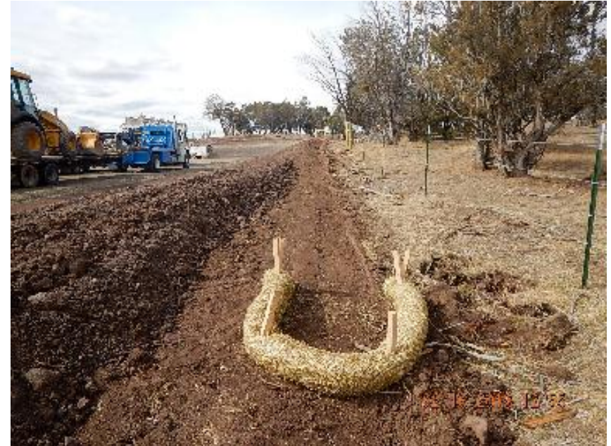
Photo 10: Check dam on N perimeter. Waddle improperly installed.
