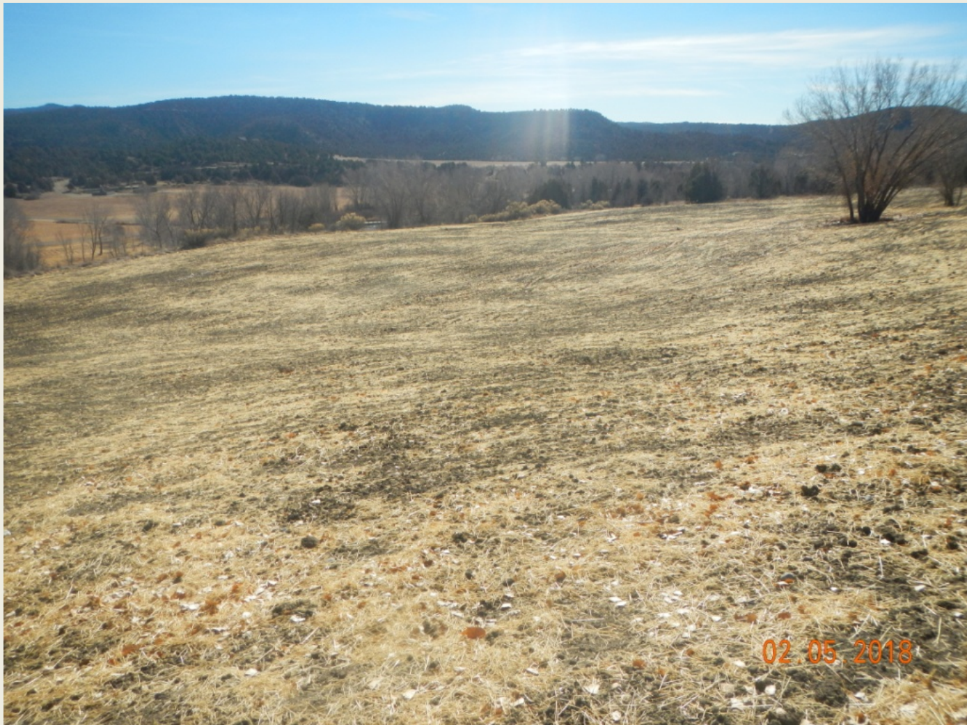
Photo 1. View of the project area from the northwestern corner facing center. Well pad and access are recontoured, appear to be seeded, and is mulched with straw mulch. Germination, weeds, stormwater, and vegetation establishment will continue to need monitoring.
