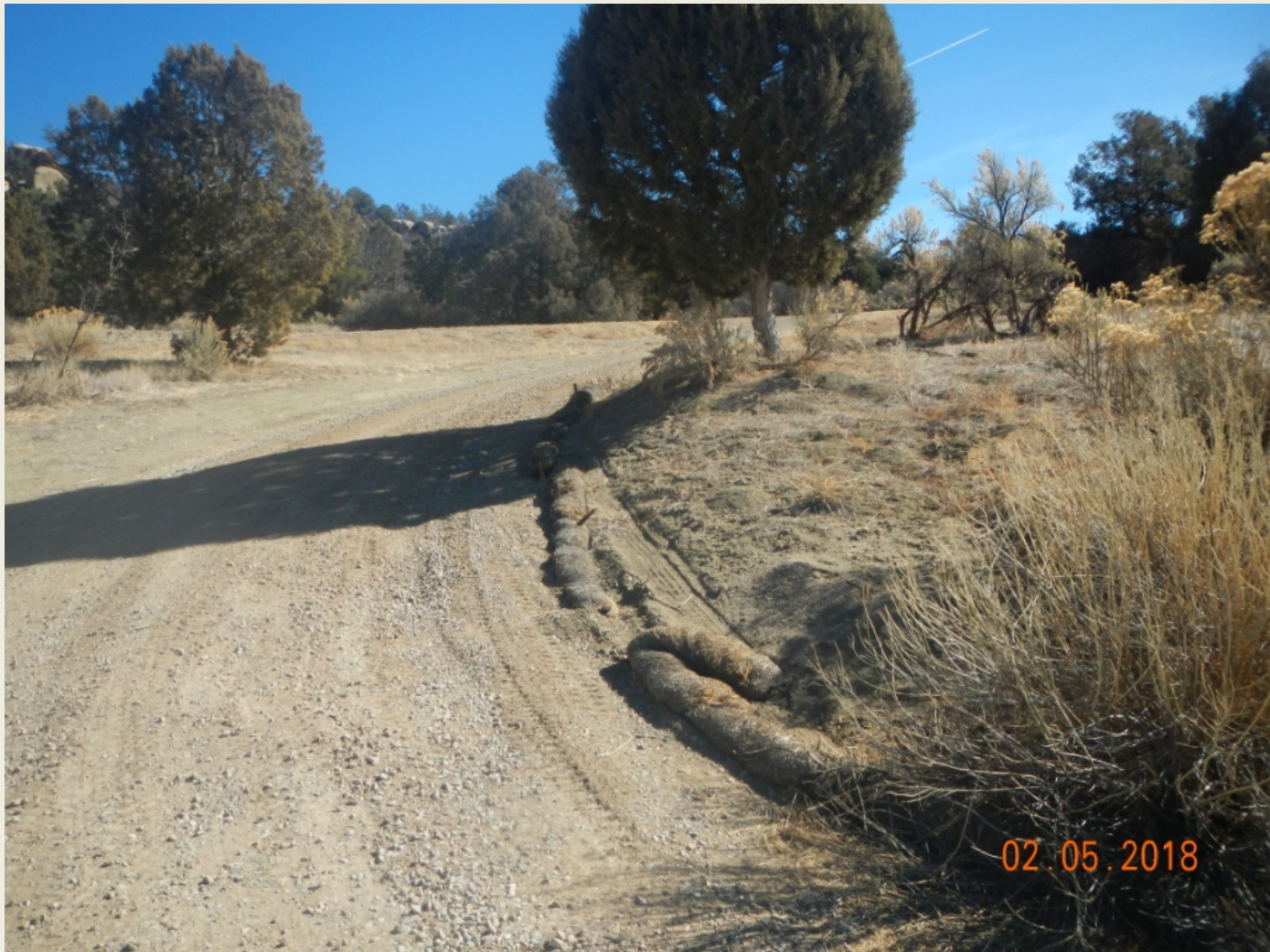
Photo 6. View of wattles on the south side of the access near the well pad entrance that need maintenance/replacement.
