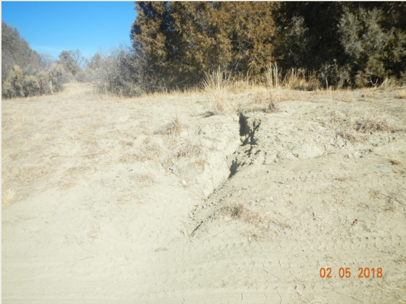
Photo 5. View of erosional channel forming in the northeastern portion of the project area.
