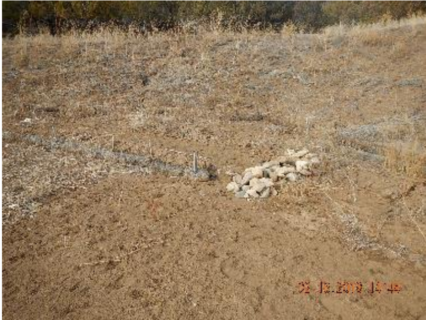
Photo 9: Check dam and waddle breach in NE corner.
