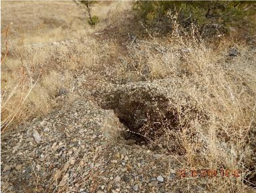
Photo 7: Erosion channel on E perimeter looking down slope.
