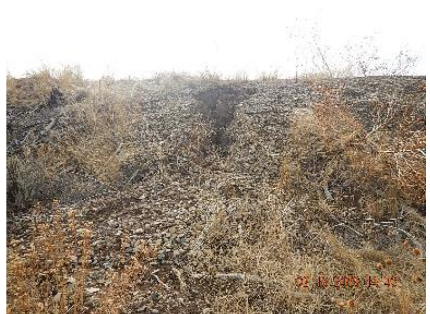
Photo 8: Erosion channel on E perimeter looking up slope.
