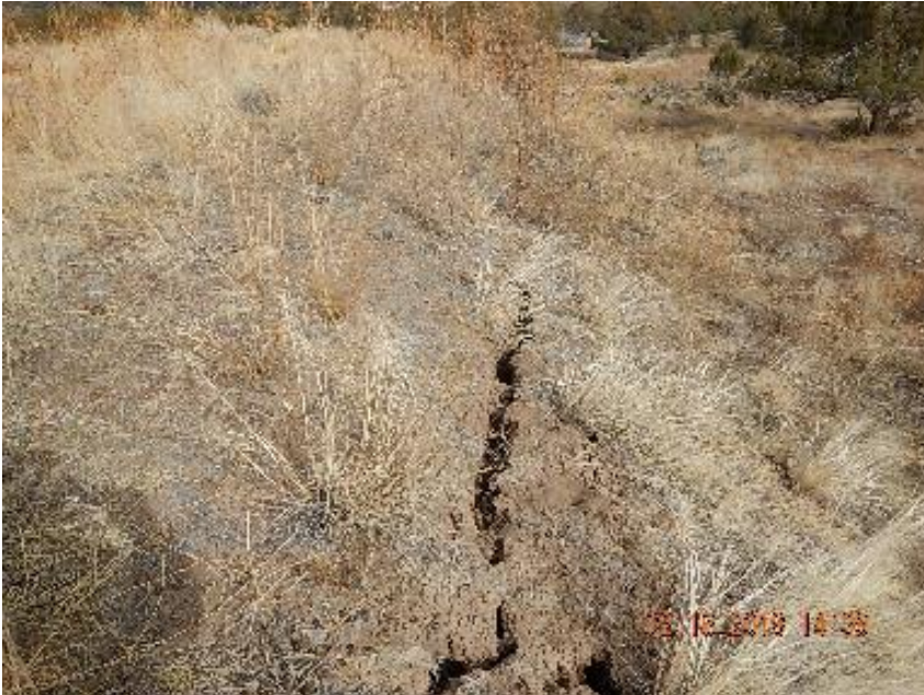
Photo 3: Soil separation at SE corner slope.
