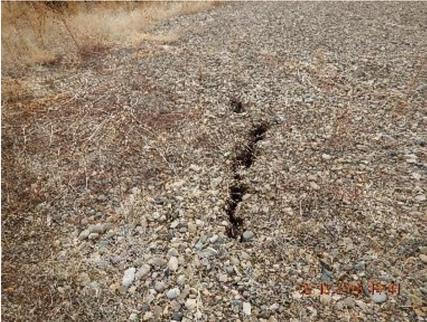
Photo 5: Soil separation at SE corner.
