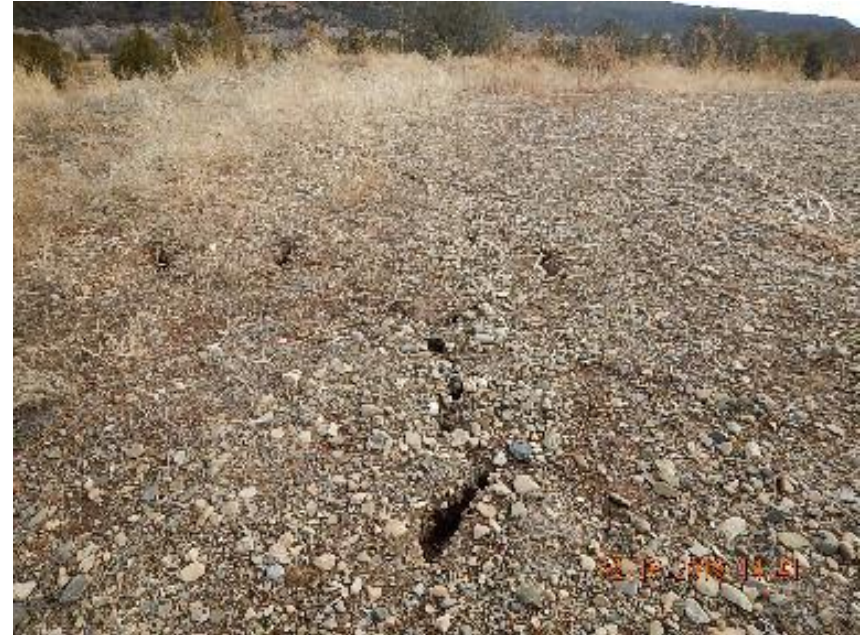
Photo 6: Soil separation at SE corner.
