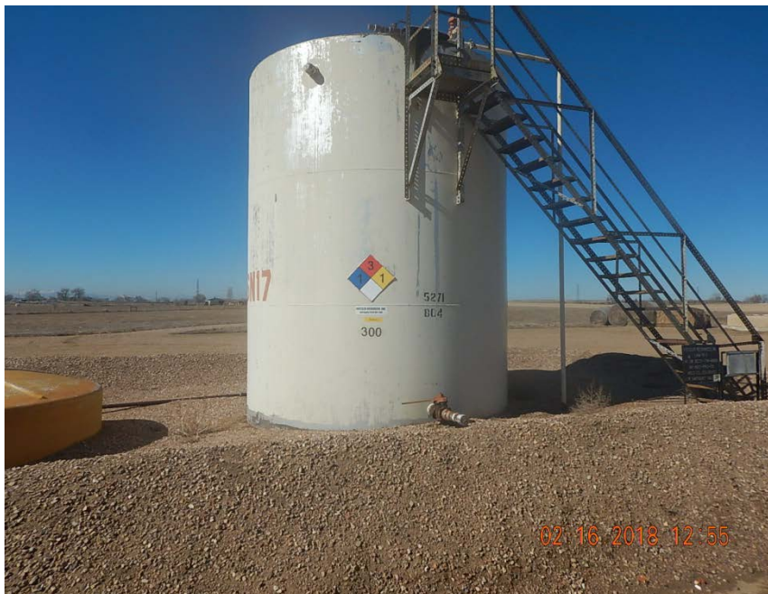
Photo 1: Location, looking NW, tank requires painting.
