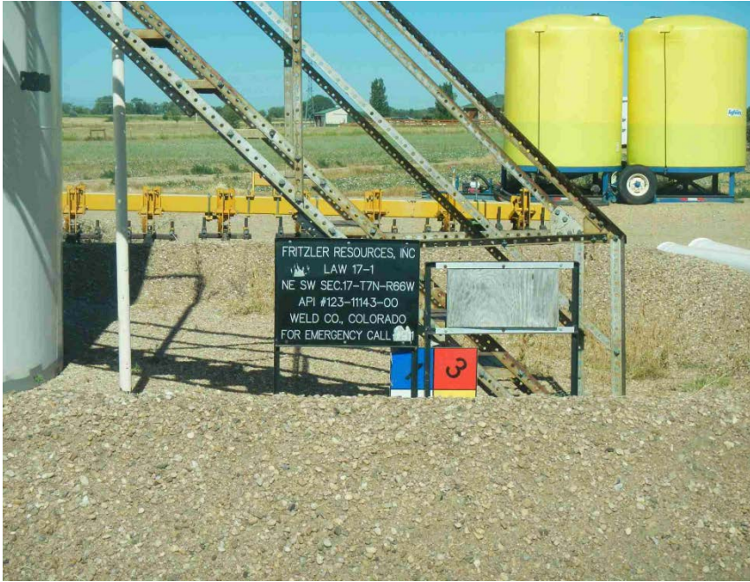
Photo from J Rickard's prior inspection for comparison
