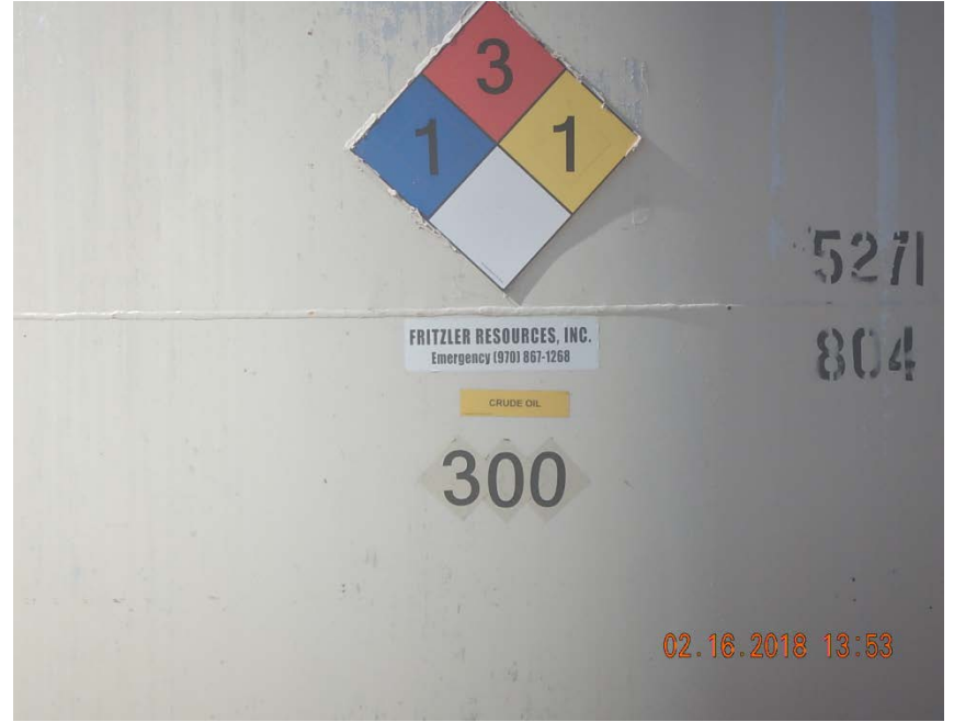
Photo 5: Emergency number decal not readable at 100 ft
