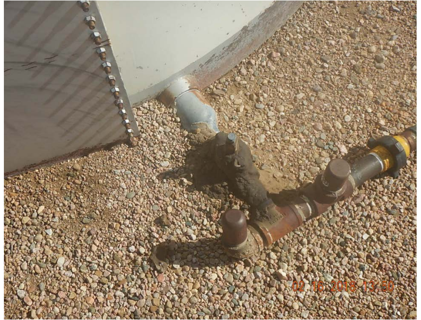
Photo 8: Stained soil at tank valve.
