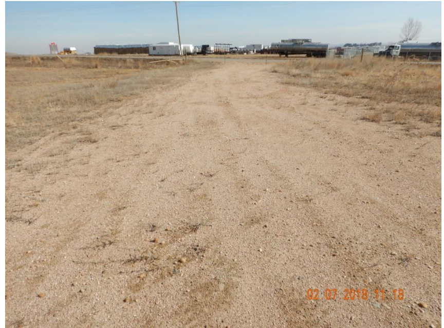
Photo 2. Photo taken from an access road off CR 53 on February 7, 2018, facing East. Operator has failed to perform final reclamation activities by the corrective action date of November 15, 2017.
