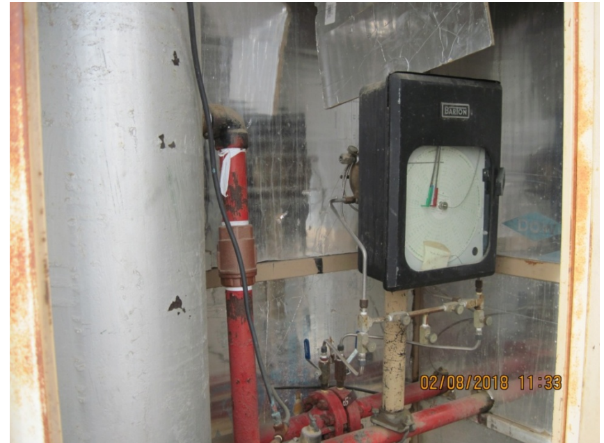
4. Monk 1-18 meter and vertical gas separator
