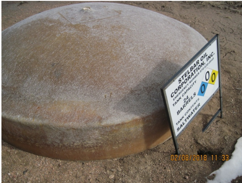
5. 24 bbl Fiberglass water tank 50% buried
