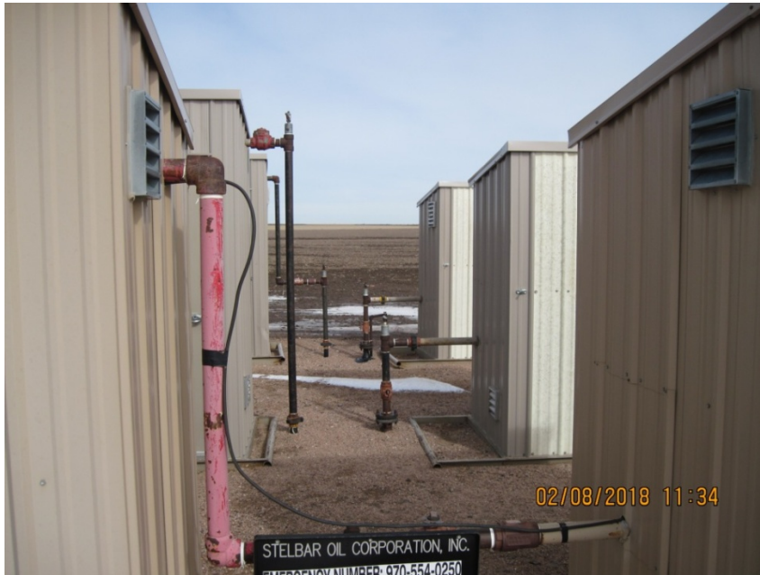
3. Central battery f/(Monk 1-18, 2-18, 3-18, 4-18) Meter sheds and Vertical gas separators in sheds
