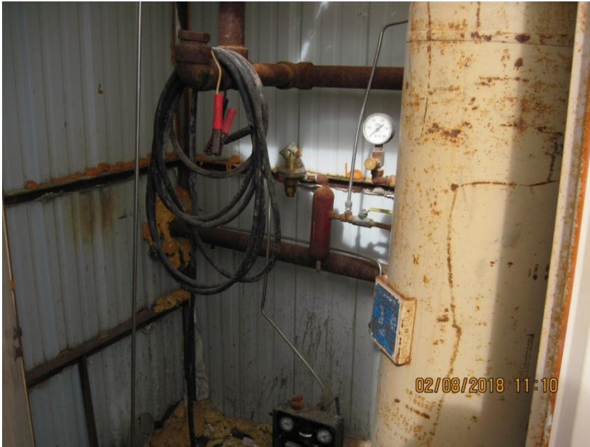
5. Vertical gas separator in shed
