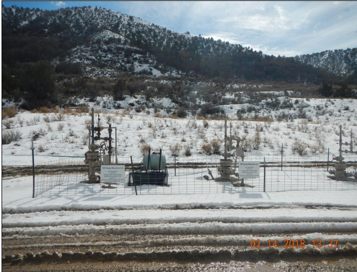
GV 52-3 well in line with newer wells on location
