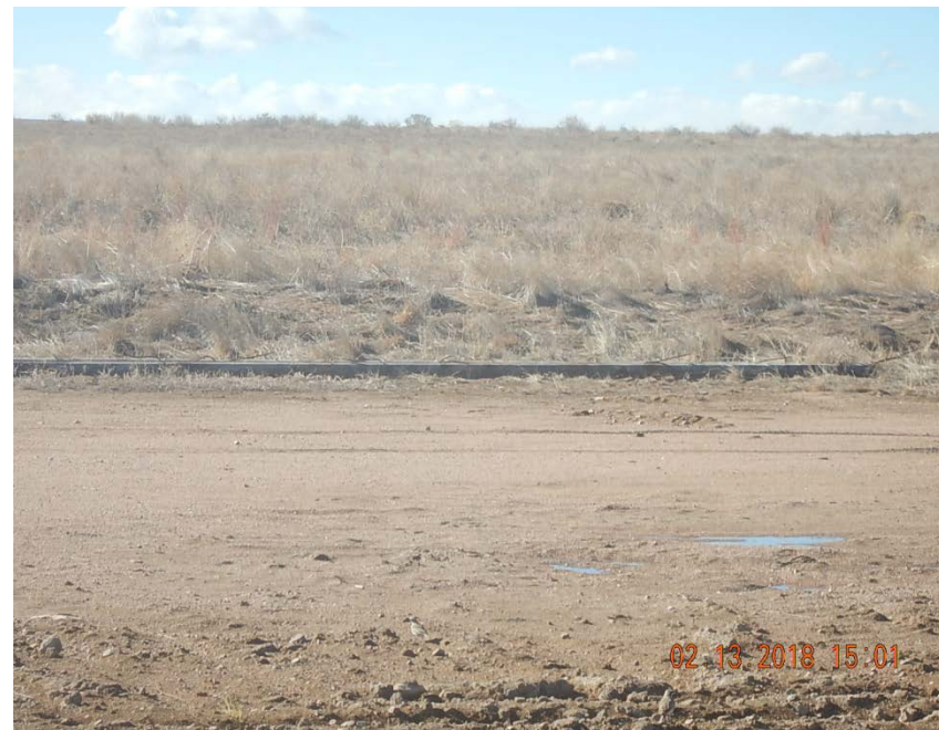
Photo 2: Unused pipe on W side of location
