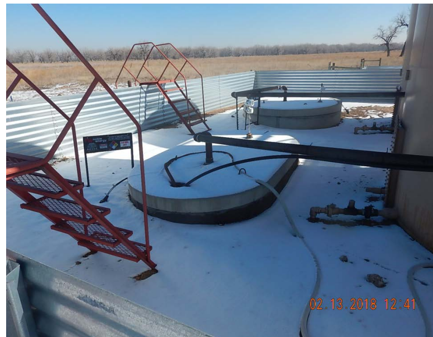
Photo 3: Vaults anchored
