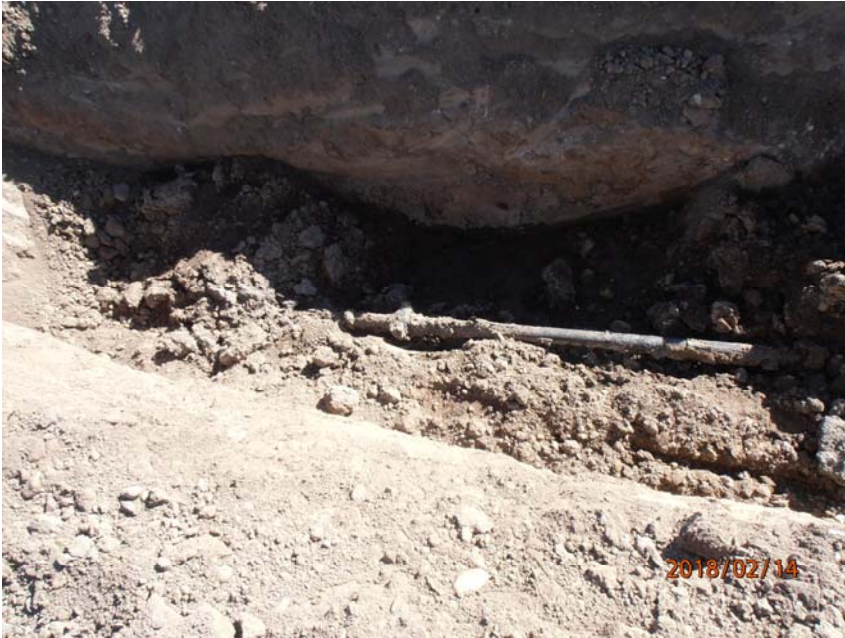
Photo 3 – Second hammer union suspected release point.
