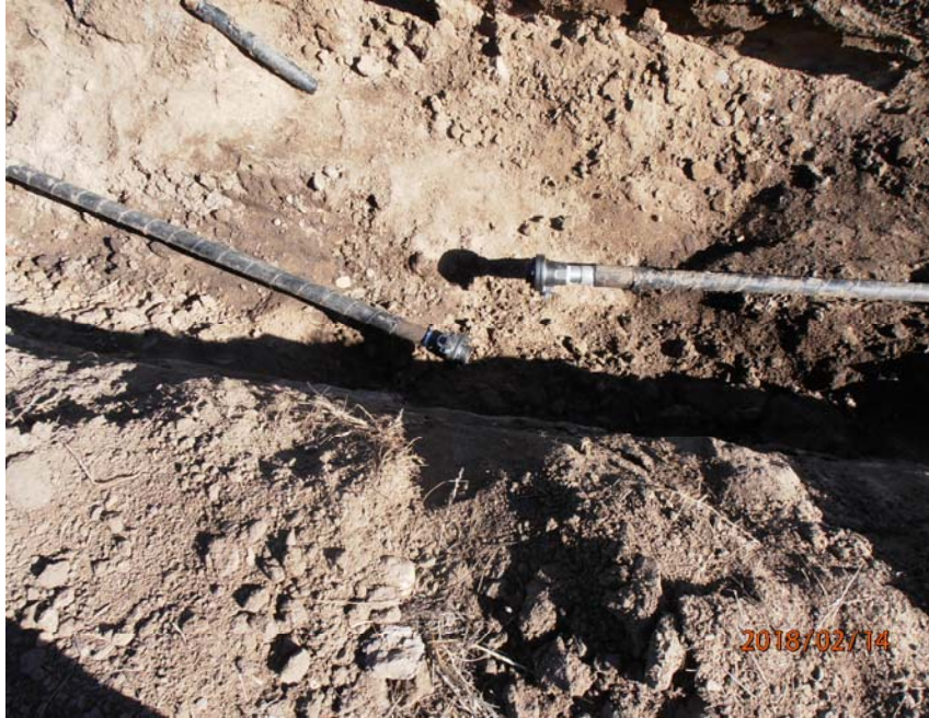
Photo 1 - Hammer union location of spill/release ID 454029
