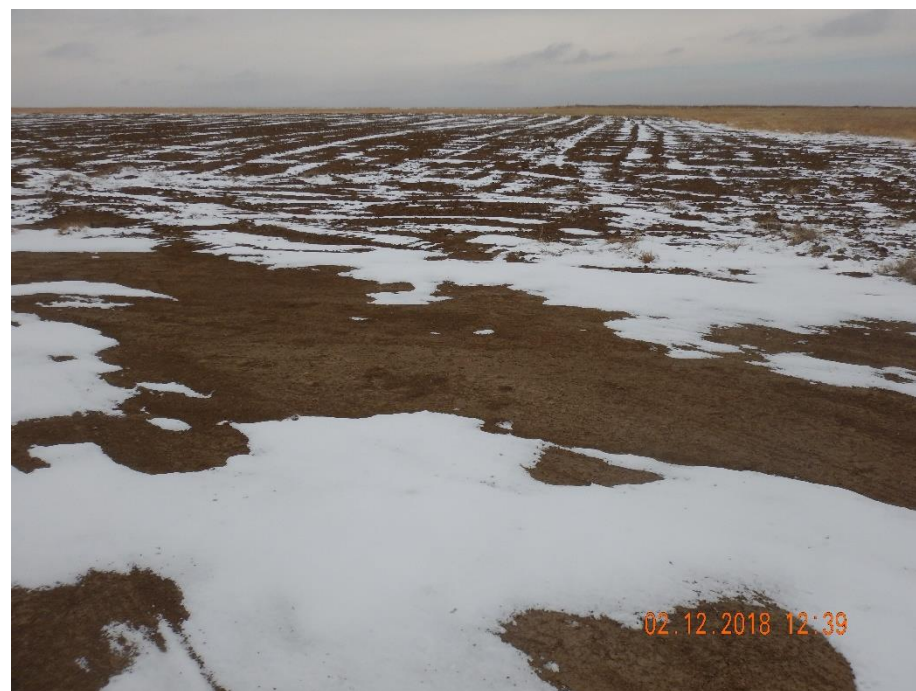
Photo 2: Photo taken from the north end of the location, facing west. Photo shows areas no longer reasonably needed for production appear to have been reduced. Topsoil appears to have been replaced. Areas appear to have been ripped for compaction alleviation. However, 1003.c requires operator to cross-rip; location appears to have only been ripped once, in one direction rather than cross-ripping. Areas within rangeland do not appear to have had revegetation activities conducted in 2017. Rig release date 8/20/2016. Interim reclamation and revegetation activities in accordance to 1003 should have been conducted by 3/20/2017.
