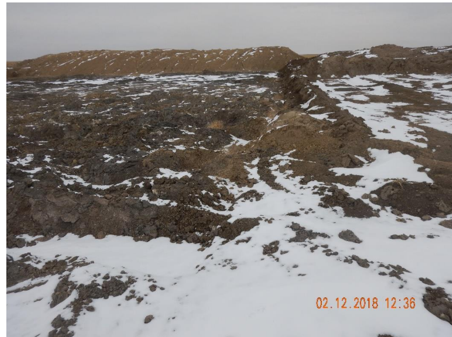
Photo 6: Photo taken from the north side of the location, facing north. Photo shows drill pit remains open. This requires closure.
