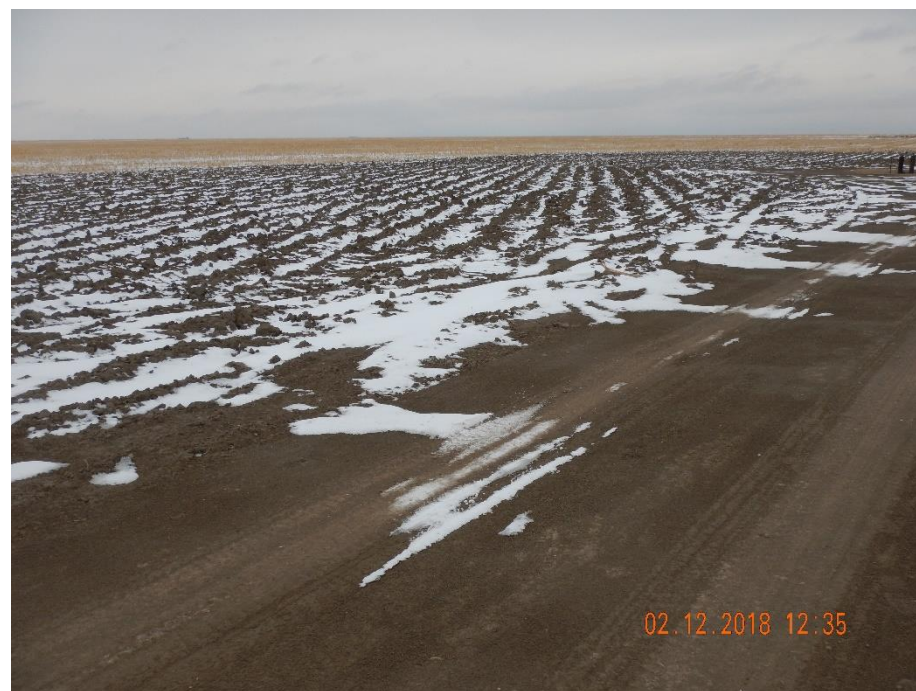
Photo 4: Photo taken from the east end of the location, facing southwest. Photo of interim reclamation in process. Photo also shows areas not reasonable needed for production have been reduced and ripped for compaction alleviation. However, 1003.c requires operator to cross-rip; location appears to have only been ripped once, in one direction rather than cross-ripping.
