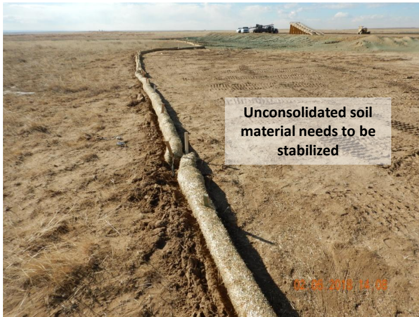
Photo 11. Photo taken from the southeast perimeter of the location on February 6, 2018, facing West. Portions of the southeastern perimeter remain unconsolidated and needs to be stabilized. Operator plans to stabilize the outer perimeter disturbance with hydromulch to prevent wind erosion.
