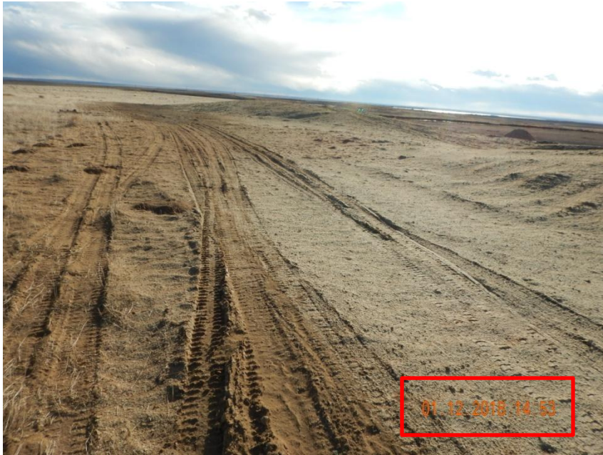
Photo 7. Photo taken from the eastern perimeter of the location on January 12, 2018, facing South. Appears the Operator has temporarily stabilized the topsoil stockpile with hydromulch. Operator does not have sufficient stormwater BMPs along the perimeter of the location.
