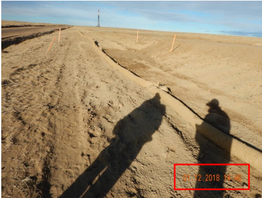
Photo 3. Photo taken from the western perimeter of the location on January 12, 2018, facing North. Straw wattle BMP has been installed and hydromulch has been applied to unconsolidated soil material along the perimeter of the location.
