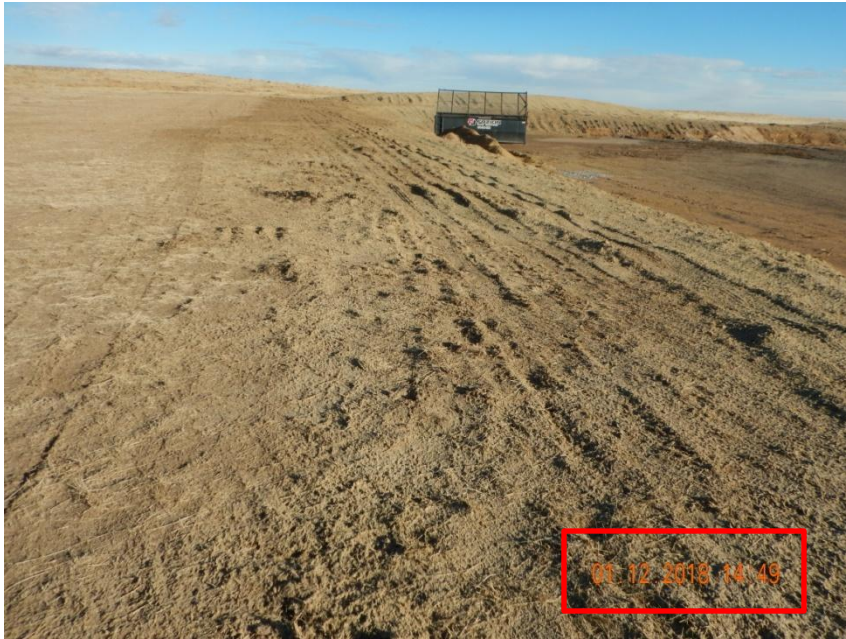
Photo 5. Photo taken from the northern perimeter of the location on January 12, 2018, facing East. Appears a surface roughening BMP has been installed along portions of the perimeter; however, this does not appear to be a sufficient and appropriate BMP for the sandy soil conditions.
