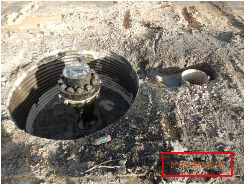
Photo 1. Photo taken from one of the wellheads at location on January 12, 2018. Photo illustrates a rat hole left open. This is a potential safety and wildlife hazard. Operator should also consider placing safety fence around the wellhead area for safety measures.
