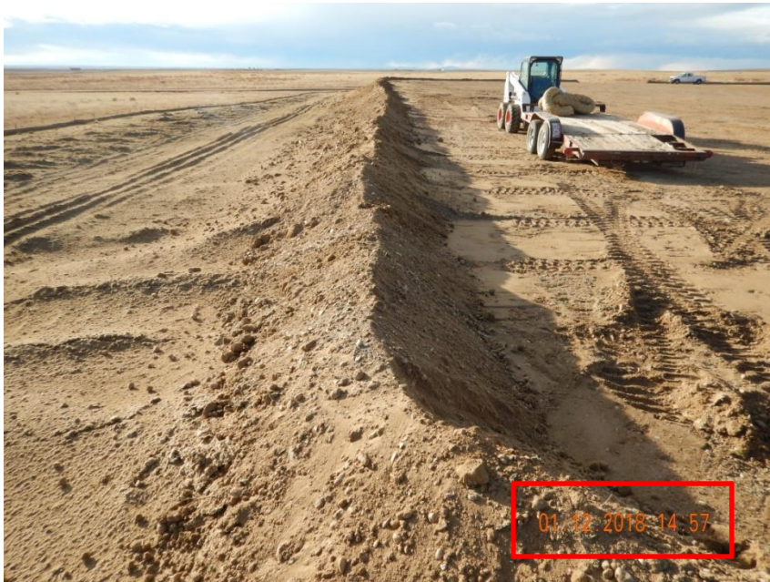
Photo 9. Photo taken from the southeastern perimeter of the location on January 12, 2018, facing West. Operator has not properly stabilized the berm BMP.
