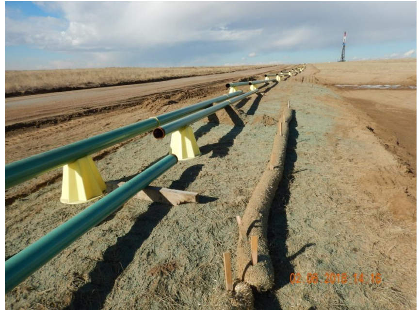
Photo 4. Photo taken from the western perimeter of the location on February 6, 2018, facing North. Pipeline installation is in-process and appears to have compromised portions of the perimeter straw wattle BMPs. Operator shall work with the Pipeline company to ensure stormwater BMPs are maintained at all times.
