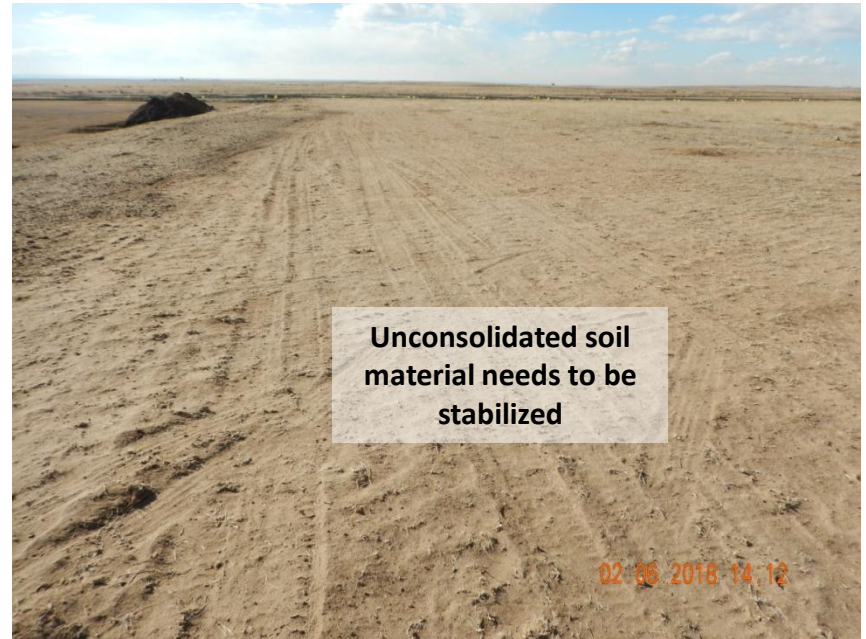
Photo 6. Photo taken from the northern perimeter of the location on February 6, 2018, facing East. Portions of the northern perimeter remain unconsolidated and needs to be stabilized. Operator plans to stabilize the outer perimeter disturbance with hydromulch to prevent wind erosion.
