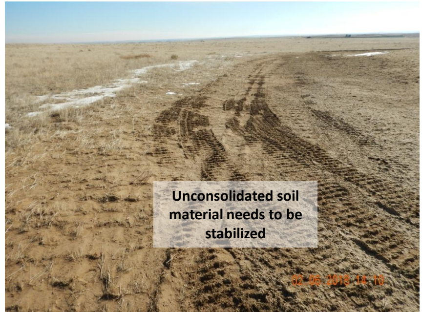
Photo 8. Photo taken from the eastern perimeter of the location on February 6, 2018, facing South. Portions of the eastern perimeter remain unconsolidated and needs to be stabilized. Operator plans to stabilize the outer perimeter disturbance with hydromulch to prevent wind erosion.
