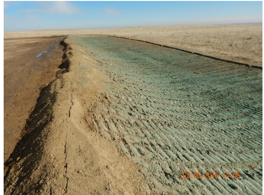
Photo 10. Photo taken from the southeastern perimeter of the location on February 6, 2018, facing East. Operator has re-tracked fill slopes, compacted the berm BMP and applied more hydromulch. Operator plans to stabilize the outer perimeter disturbance with hydromulch to prevent wind erosion.
