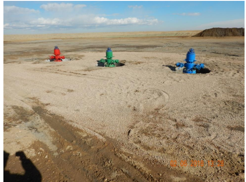
Photo 2. Photo taken from the wellheads at location on February 6, 2018. Operator has backfilled rat holes.
