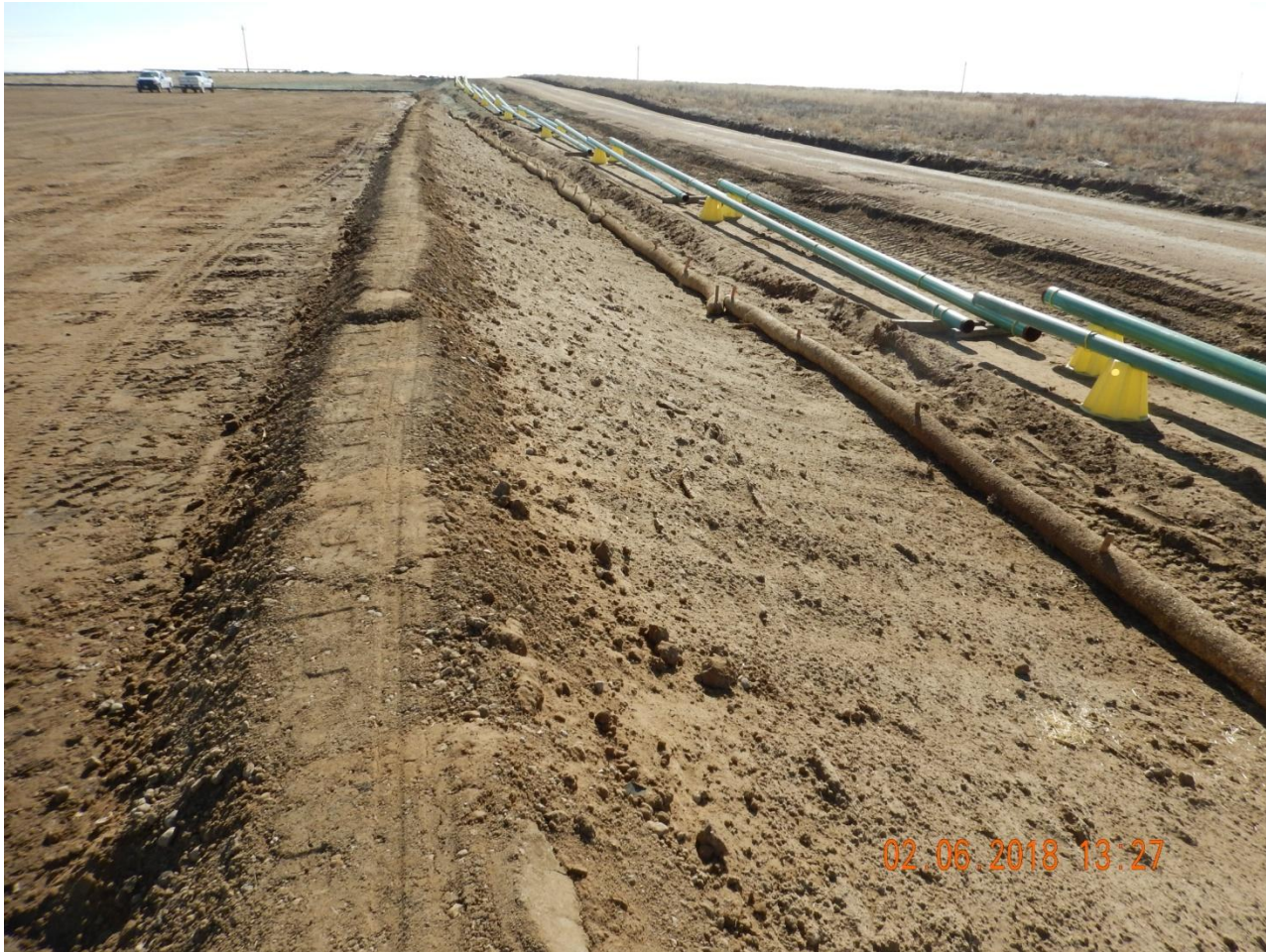
Photo 9. Photo taken from the western perimeter of the location on February 6, 2018, facing South. Pipeline installation is in-process and appears to have compromised portions of the perimeter straw wattle BMPs. Operator shall work with the Pipeline company to ensure stormwater BMPs are maintained at all times.
