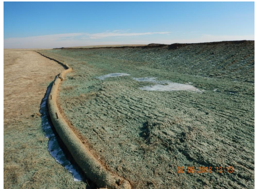
Photo 8. Photo taken from the northwest perimeter of the location on February 6, 2018, facing East. Operator has re-tracked fill slopes and applied more hydromulch. Operator plans to stabilize the outer perimeter disturbance with hydromulch to prevent wind erosion.
