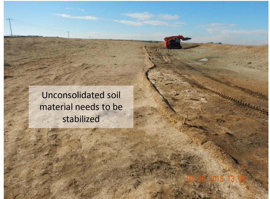
Photo 4. Photo taken from the southeastern perimeter of the location on February 6, 2018, facing West. Portions of the southern perimeter remain unconsolidated and needs to be stabilized. Operator plans to stabilize the outer perimeter disturbance with hydromulch to prevent wind erosion.
