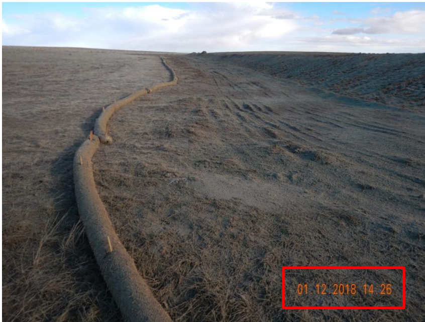
Photo 7. Photo taken from the northwest perimeter of the location on January 12, 2018, facing East. Straw wattle BMP has been installed and appears hydromulch has been applied to portions of unconsolidated soil material along the perimeter of the location.
