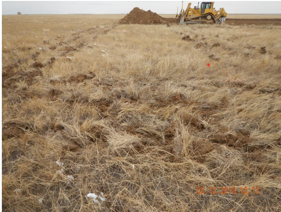
Photo 3: Photo shows operator expanded surface roughening BMPs as needed to better suit the size of the location during construction activities.
