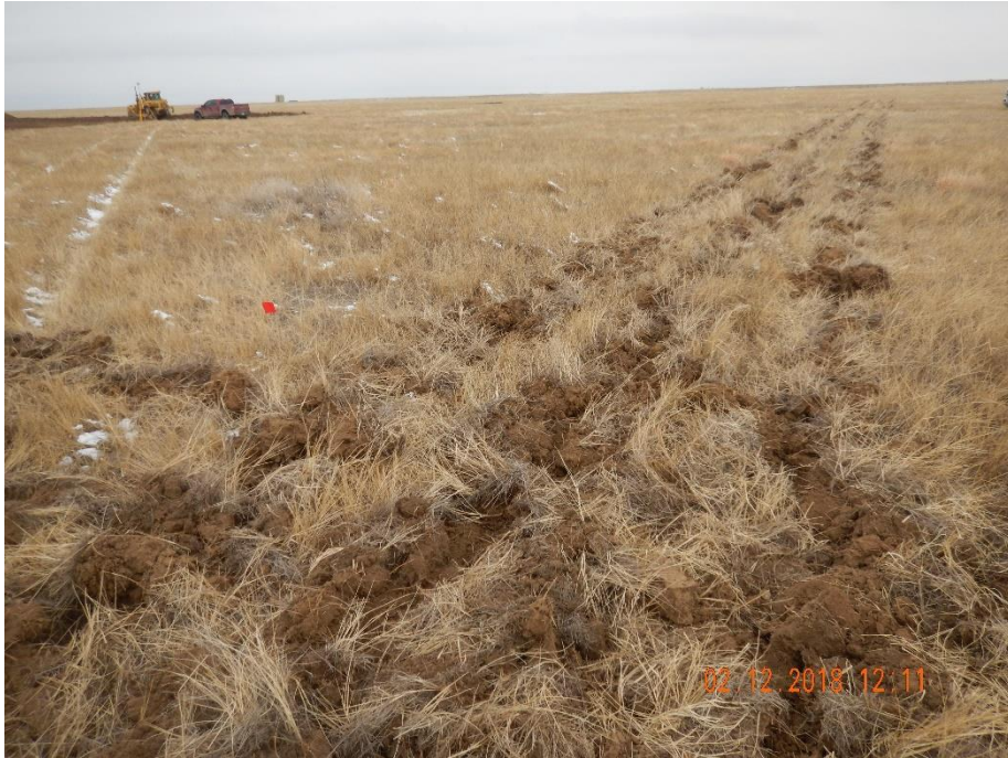
Photo 1: Photos 1-10 show surface roughening stormwater BMP implemented along the perimeter of the location prior to construction activities.
