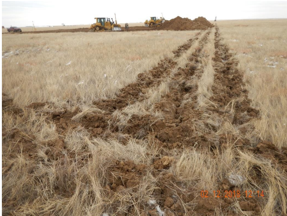
Photo 5: Operator was in the process of salvaging topsoil at time of inspection.
