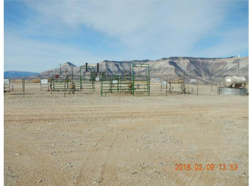
Looking north. Fenced wellheads. Horizontal tank is labeled and has secondary containment. No stains, no junk. No vegetation observed in this area.
