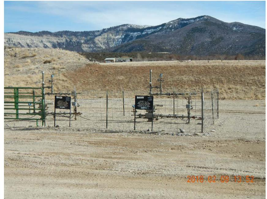
Wellheads fenced and labeled. No staining or fluids observed around the wellheads.
