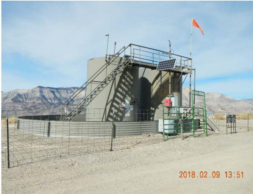
Produced and condensate 300 bbl tanks. Lined, bermed and fenced. Signs with emergency and wells information. A sign warning of potential H2S is posted on the tanks.
