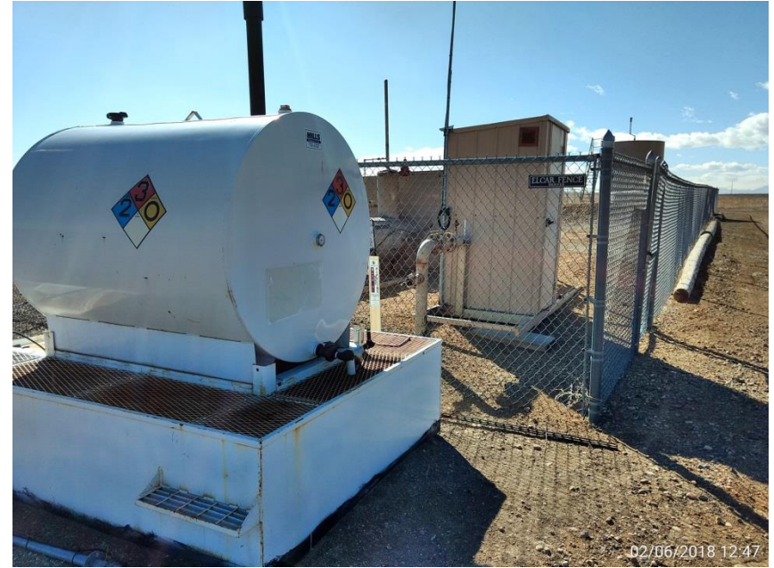
Appears to be unused chemical tank. Corrective Action: Unused equipment, address per rule 603.f
