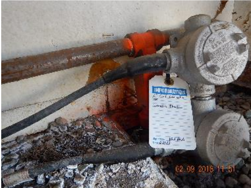
Photo 3: Unused riser. Plugged, painted, and tagged.
