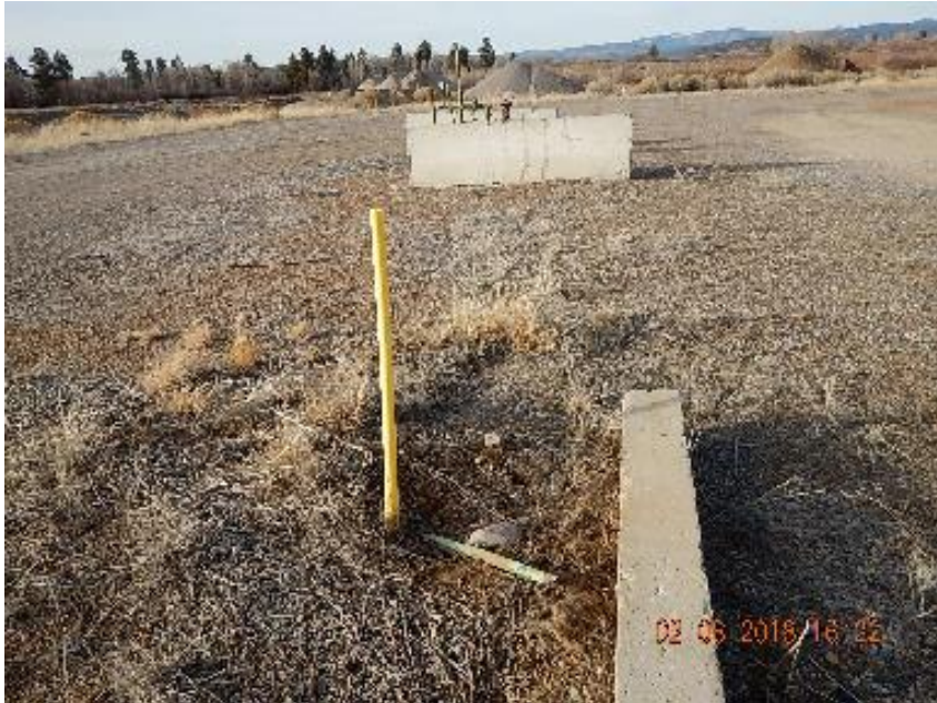
Photo 3: Bent over 1" riser S of wellhead. Line is open ended.
