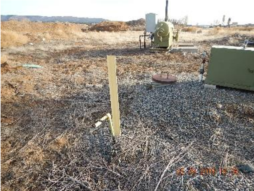
Photo 5: 1" steel riser in E perimeter of location. Valve is painted and plugged.
