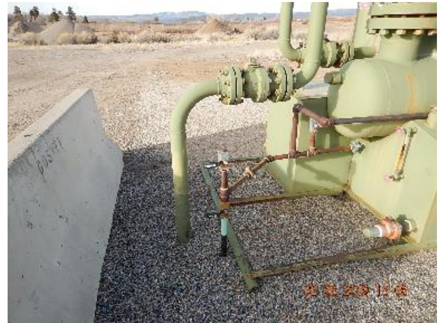
Photo 2: Unused 1" supply gas line at separator.
