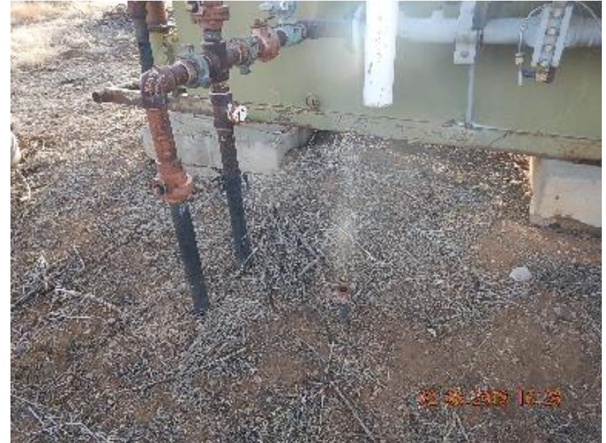
Photo 4: Unused 1" steel riser on E side of domestic tap separator. Line is open ended.
