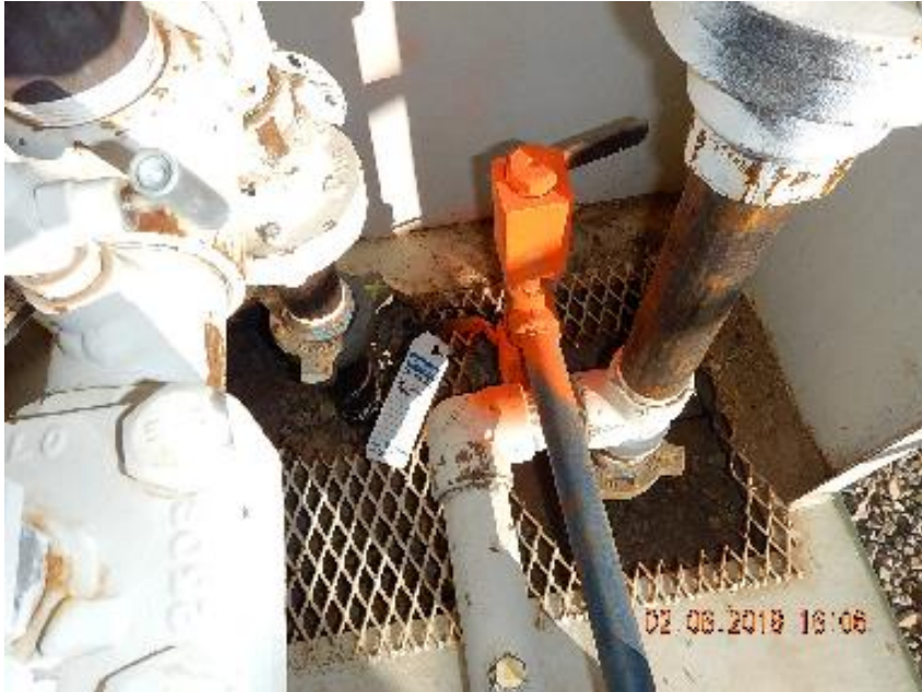
Photo 3: Unused supply gas line inside G#4 separator cabinet.
