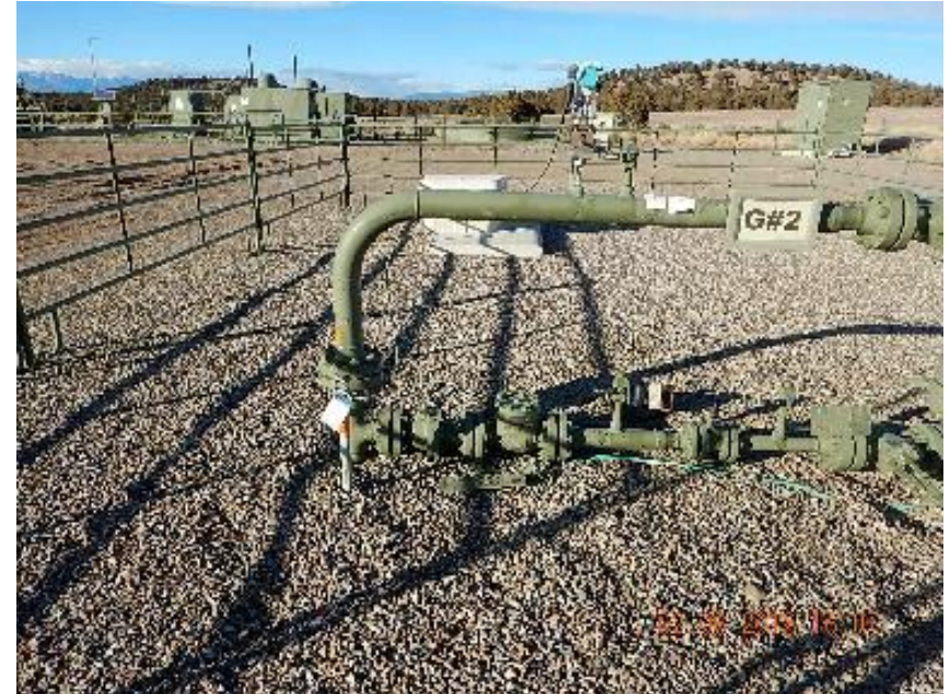
Photo 4: Unused supply gas riser at G#2 wellhead.
