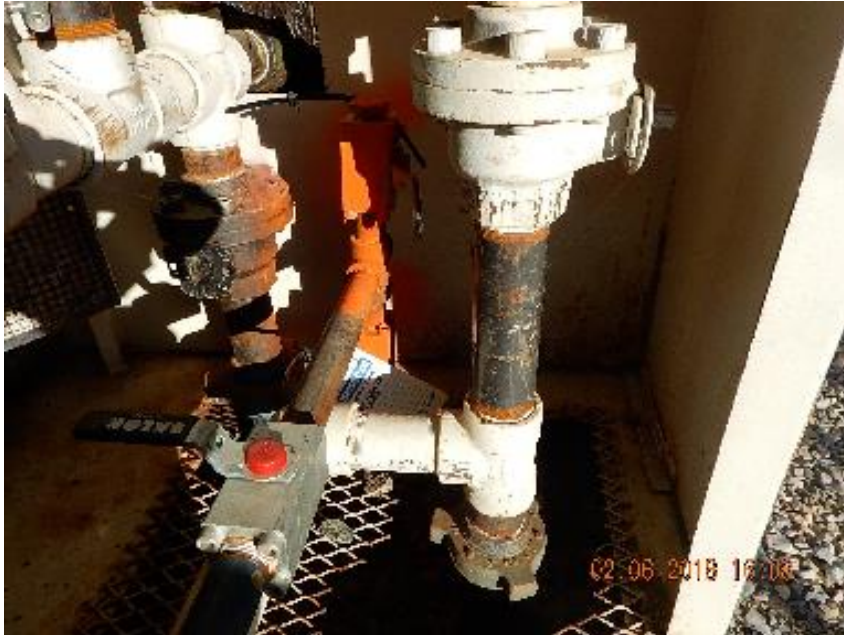
Photo 5: Unused supply gas line inside G#2 separator cabinet.
