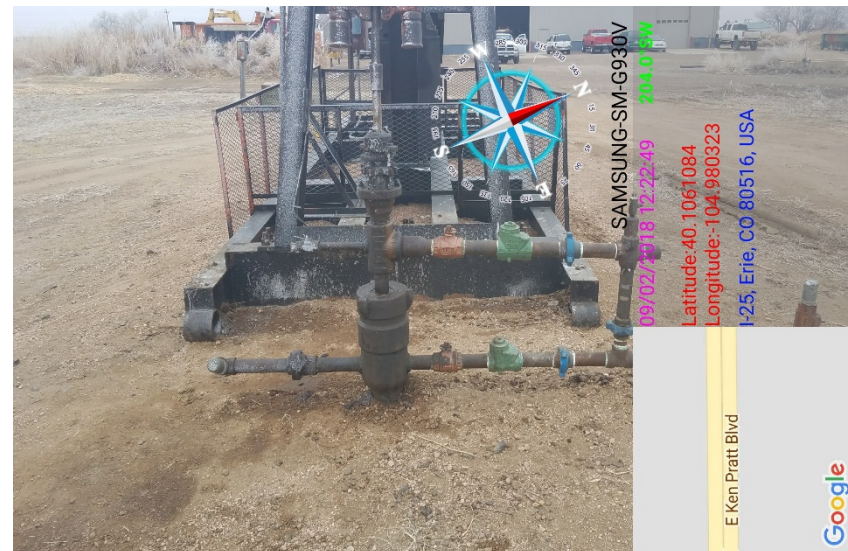
Stained soil from leaks
