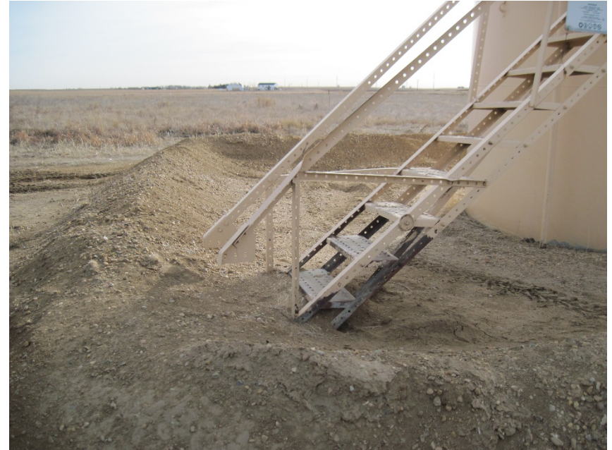
BERMS NEED REBUILT
