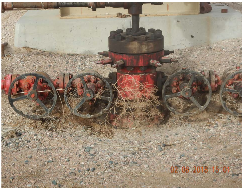
Photo 3: Stained soil at wellhead
