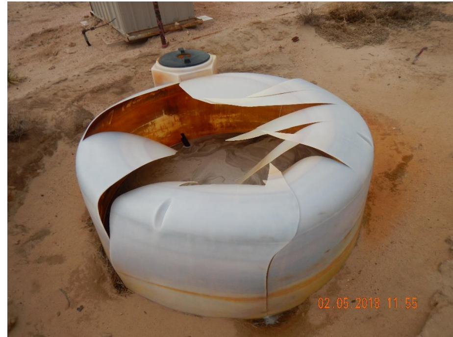
Photo 2: Photo taken from the east end of the pit. Photo shows tank in disrepair.
