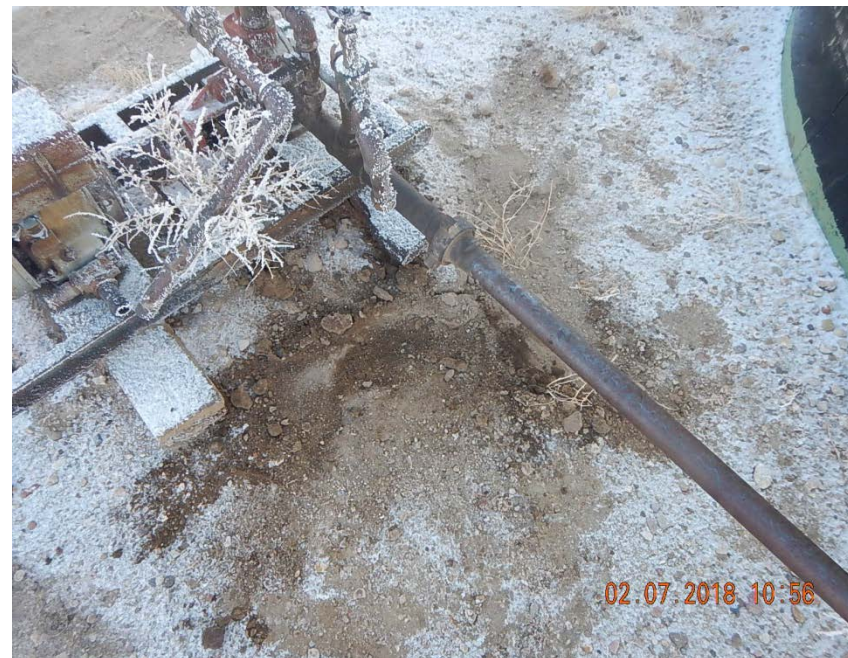
Photo 8: Stained soil at transfer pump
