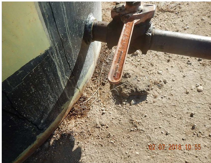
Photo 13: Stained soil at base of tank at loadout
