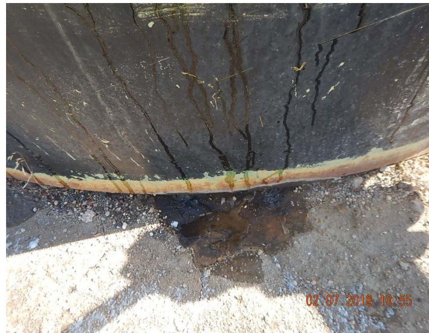
Photo 14: Stained soil and fluid at base of tank on NW side
