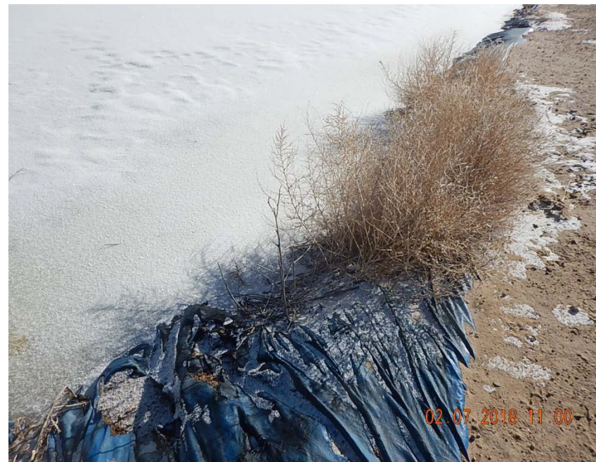
Photo 7: Pit 2 liner, torn and compromised by vegetation
