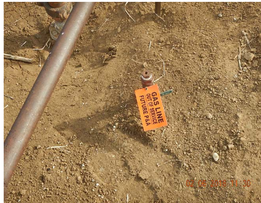
Photo 4: Riser tagged as inactive.
