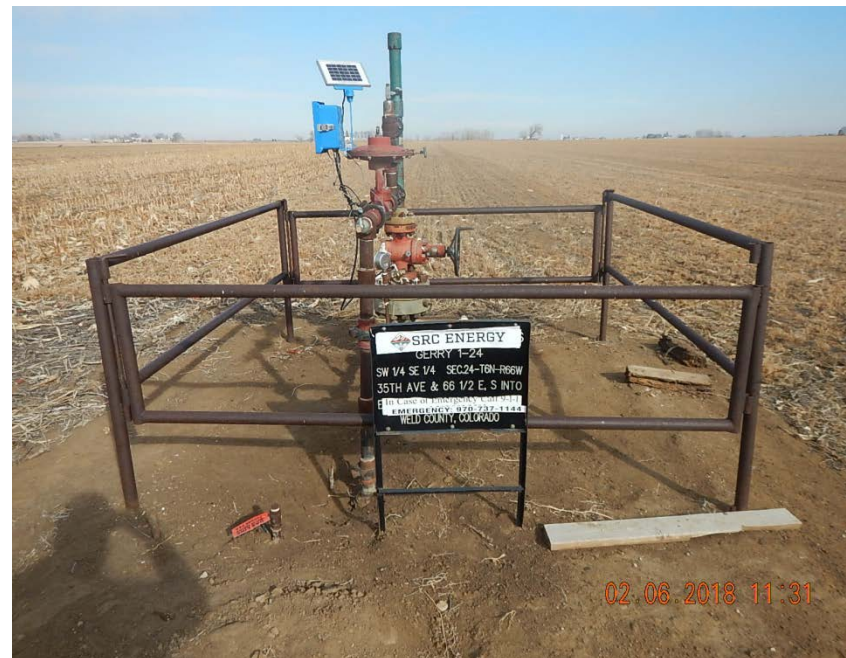
Photo 2: Wellhead, looking N
