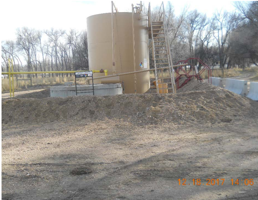
Photo from S O'Donnell's prior inspection for comparison
