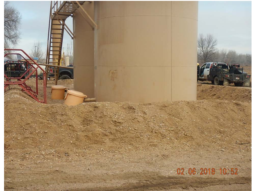
Photo 4: Berms still damaged
