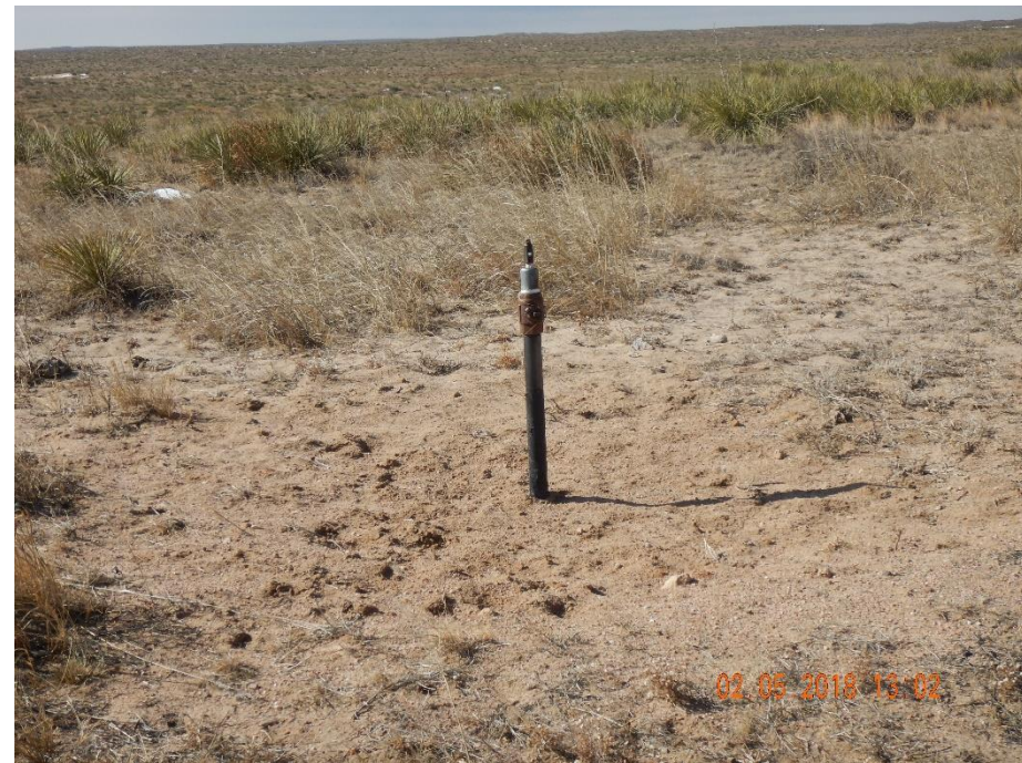
Photo 8: Photo taken access road northeast of the location at coordinates 39.83686/-102.85993. Photo shows pipe riser that has not been removed.
