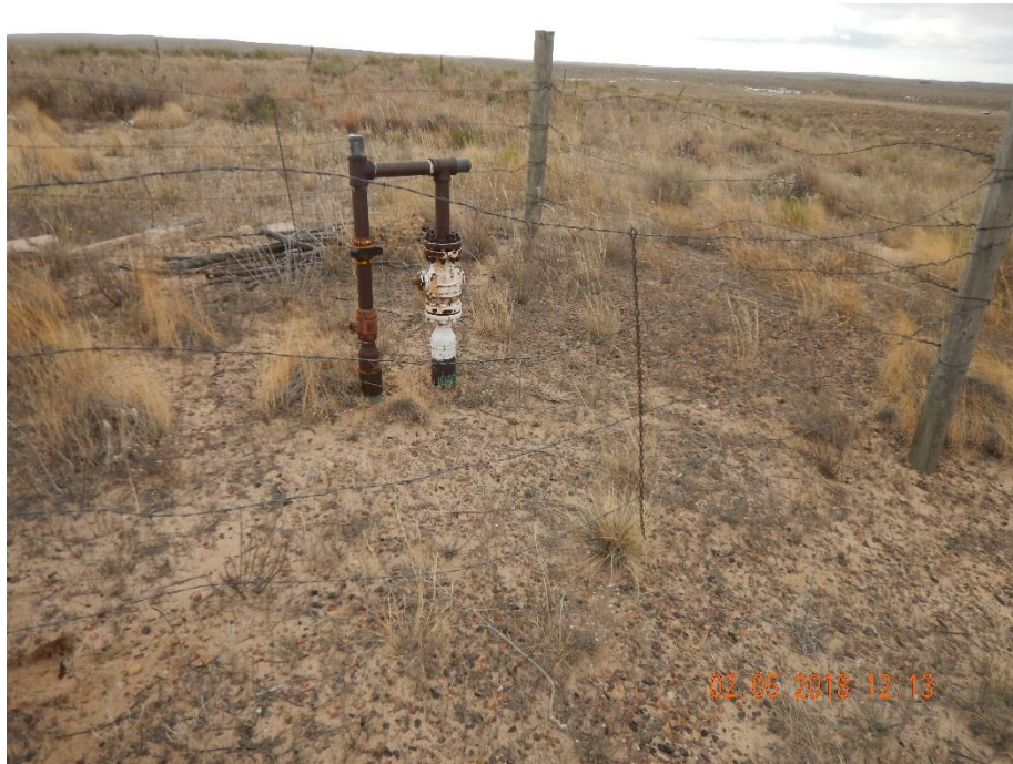
Photo 9: Photo taken from the southeast end of the location, facing south. Photo shows pipe riser, fence and debris remains on the location. Equipment was identified as a "Gasline tie/well" in previous inspection.
