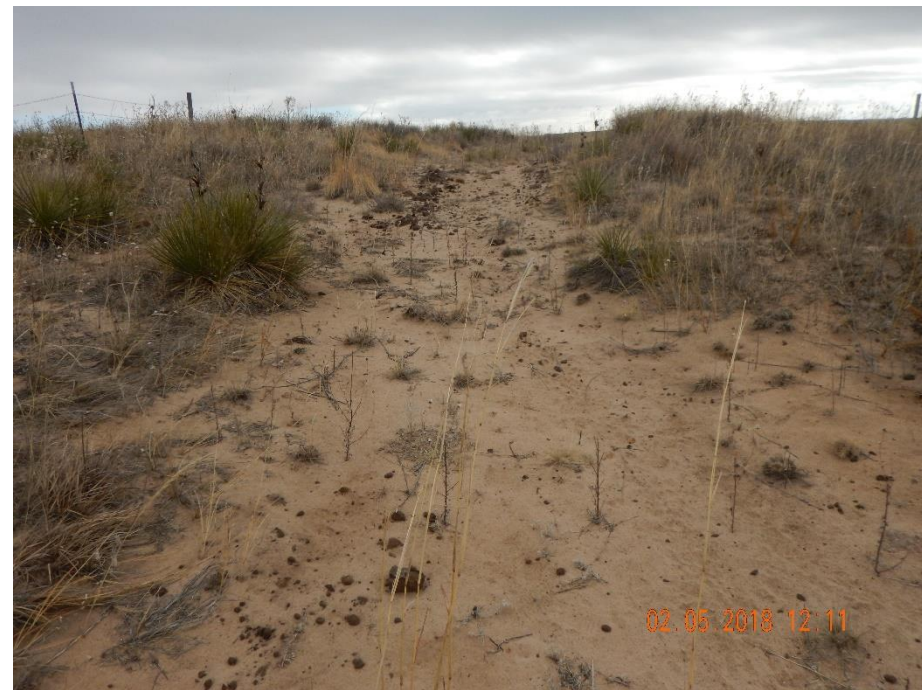
Photo 4: Photo taken the east end of the location, facing south. Photo shows portions of the access road on location have not been reclaimed per reclamation rules. Erosion evident. Dark, stained/contaminated soils have not been removed.
