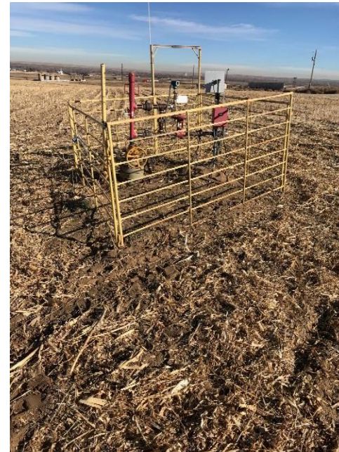
Wellhead clear of weeds after CA completed
