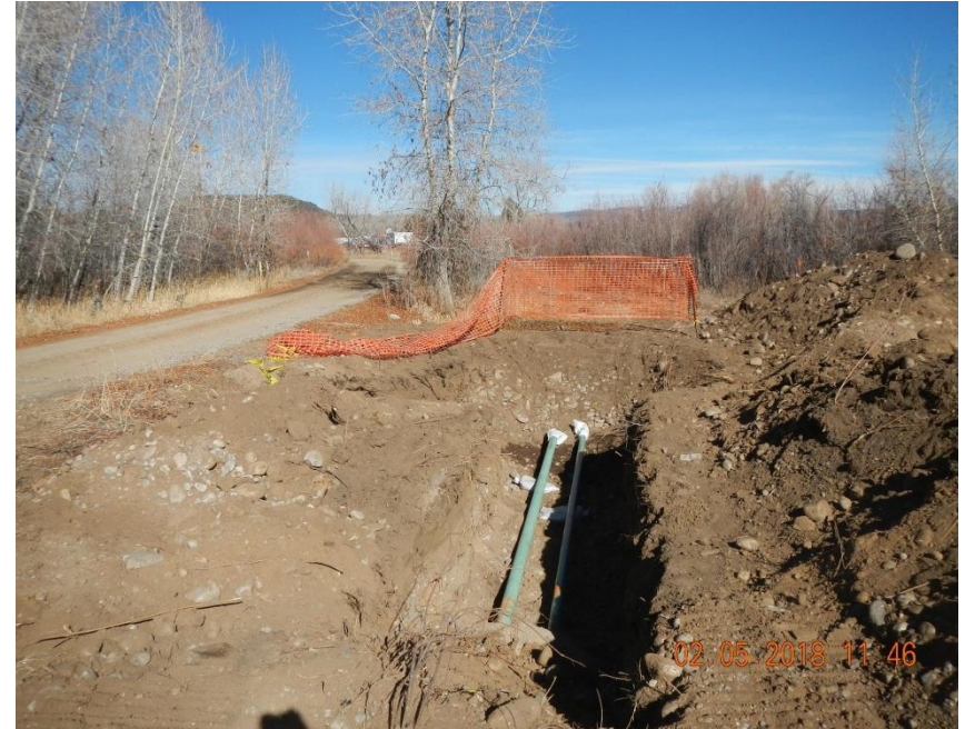
Gathering line excavation. Le Platt B #2 in background.
