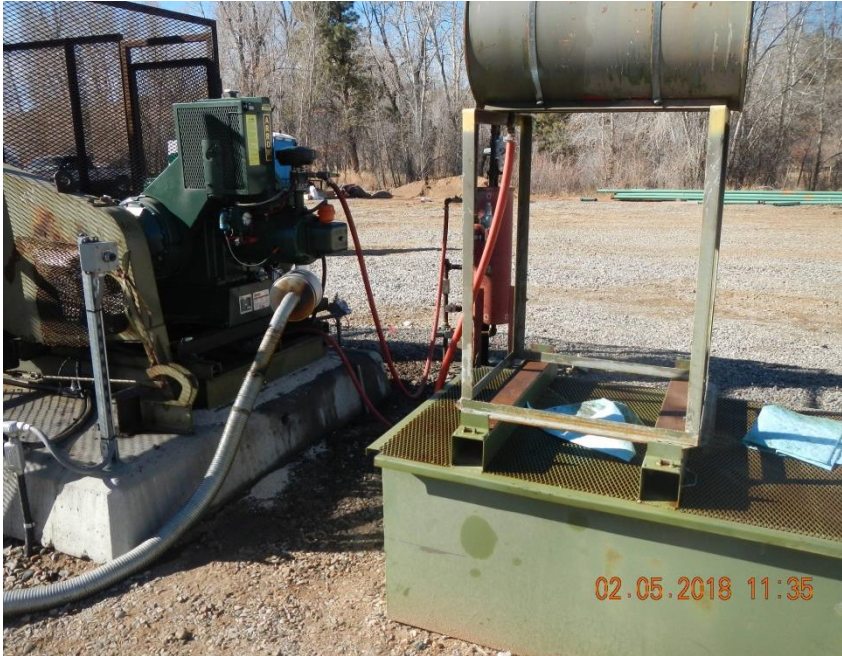
Secondary containment for lube oil container.
