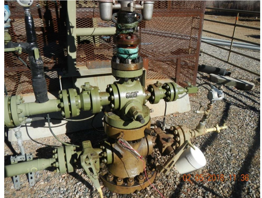
Absorbent rags on well head are saturated.
