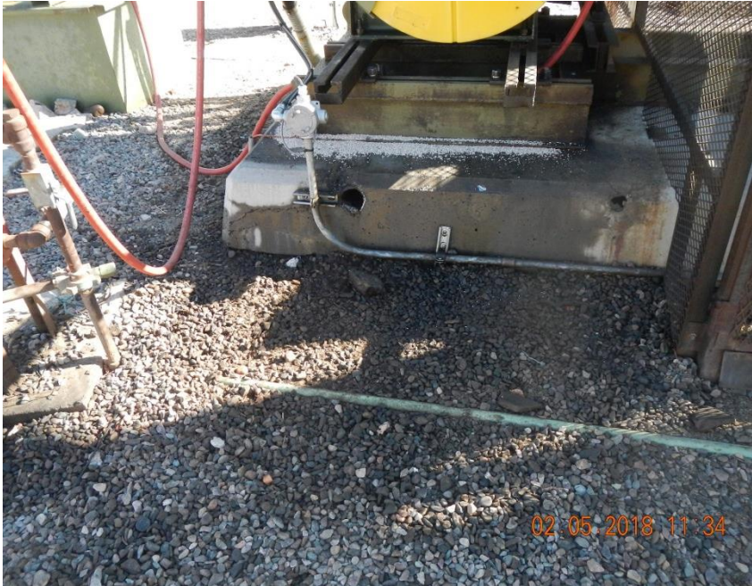
Stained concrete pad and surrounding gravel around prime mover.
