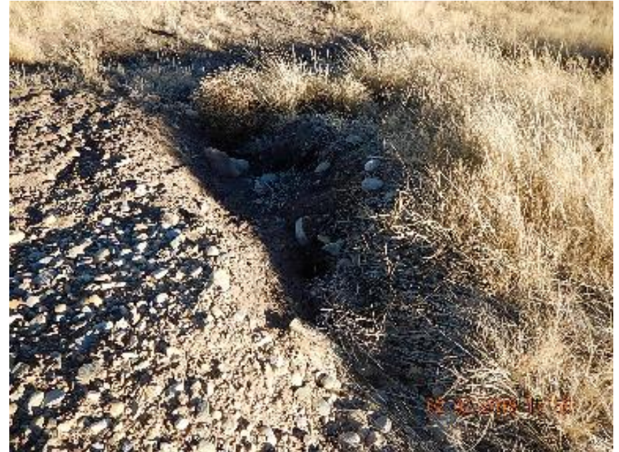
Photo 2: Erosion channel along base of tank berm.
