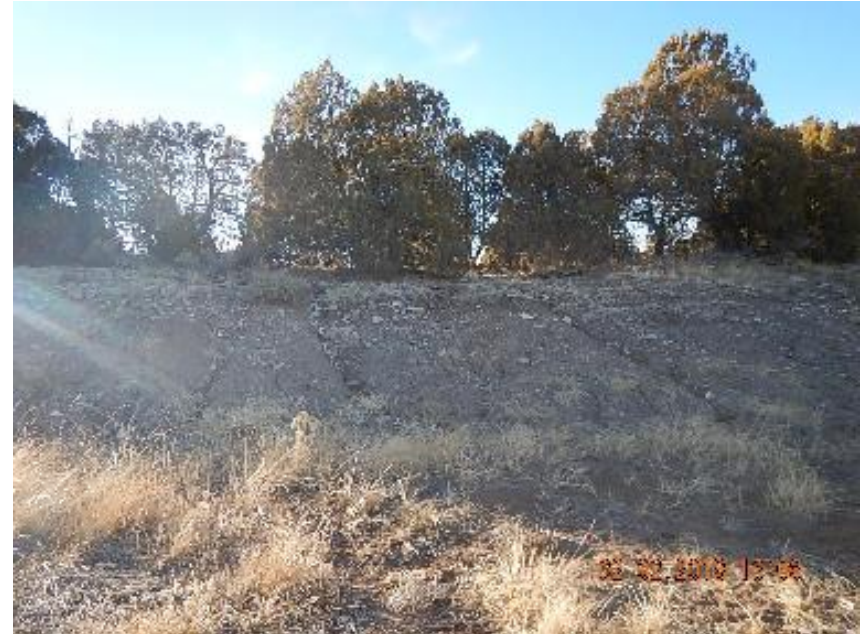
Photo 4: Erosion channels and rilling on cut slope.
