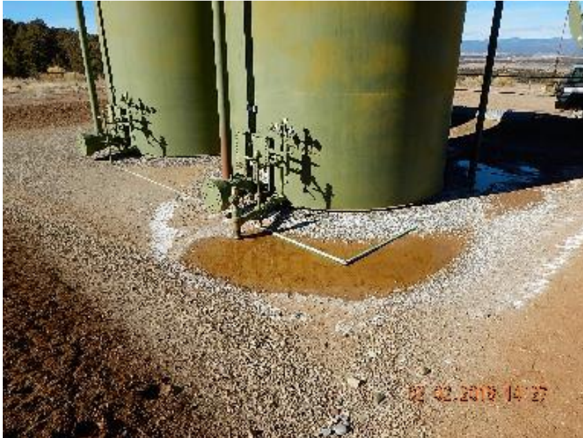
Photo 7: Mineral ring around base of tank. Inside berms.
