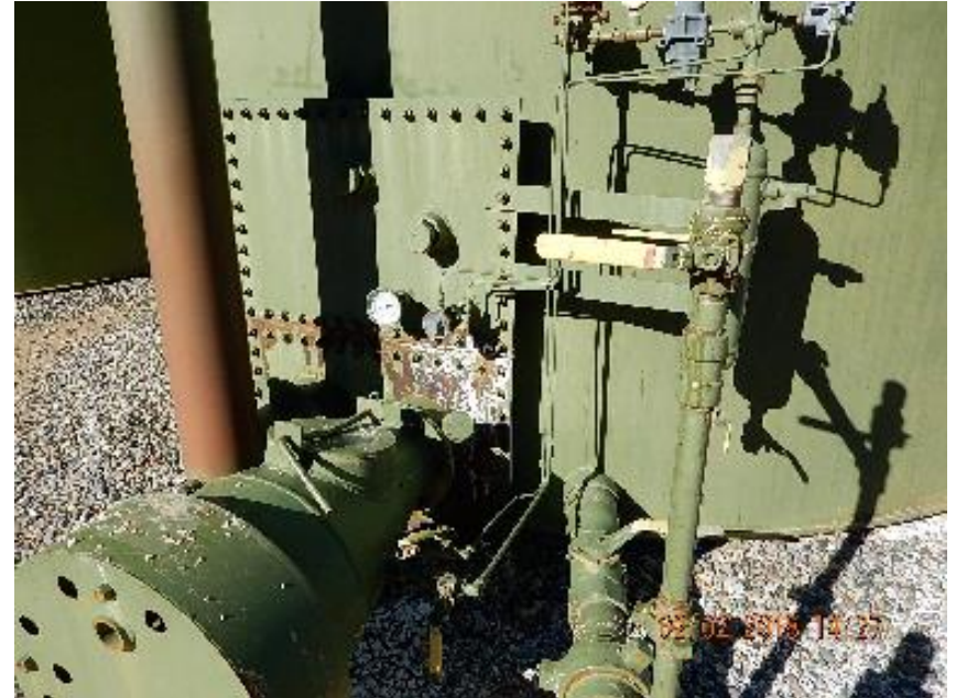
Photo 6: Mineral deposits on tank heater tube hatch.
