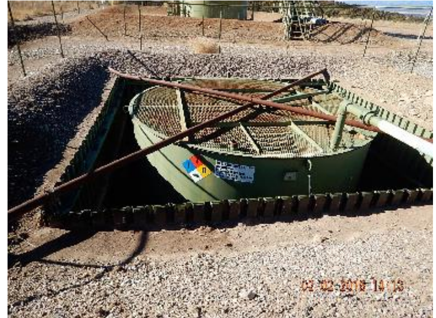
Photo 2: Open top tank with below grade labels.
