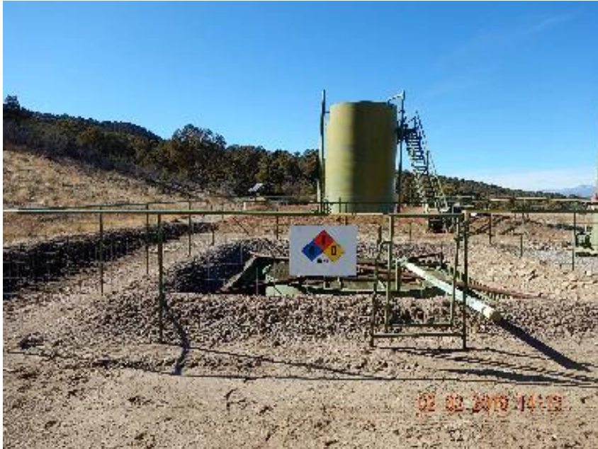
Photo 3: Tank labels below grade and not visible. NFPA label on fencing does not match label on tank.
